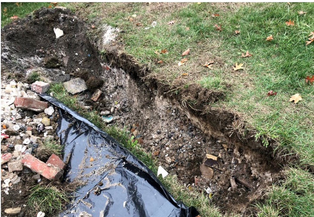
Picture 4: Test pit excavation heavily impacted with ABG.
