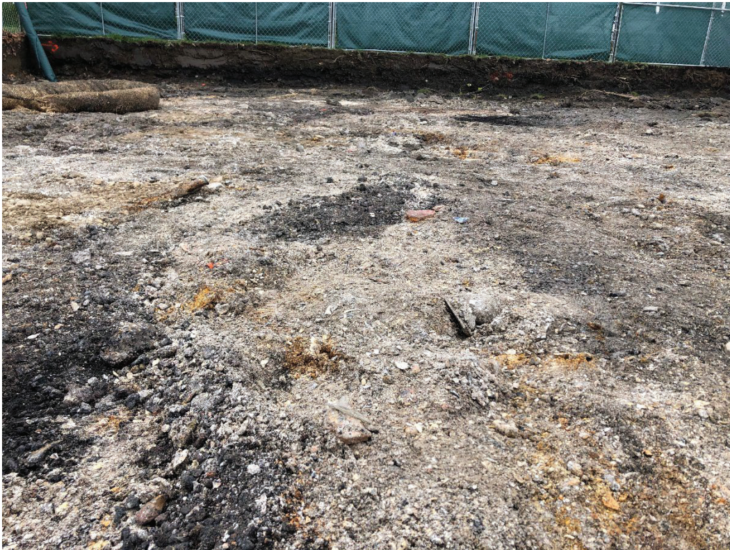
Picture 3: Excavation heavily impacted with ABG.
