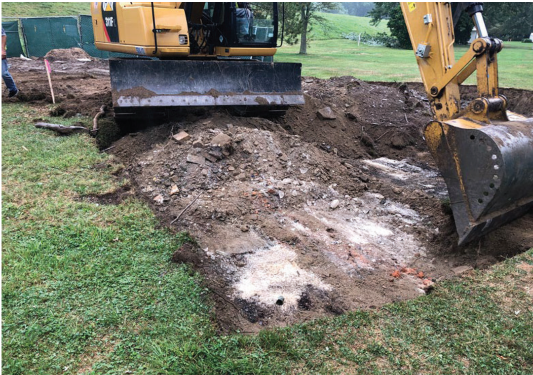
Picture 2: Excavation heavily impacted with ABG.
