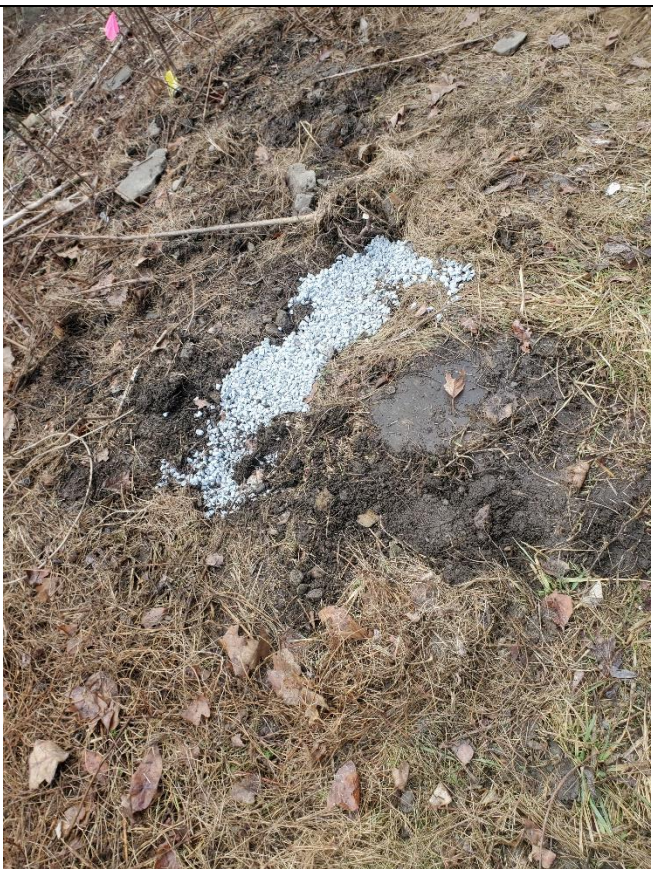
Picture 4 View looking Southwest: Bentonite chip backfills at SS-07.
