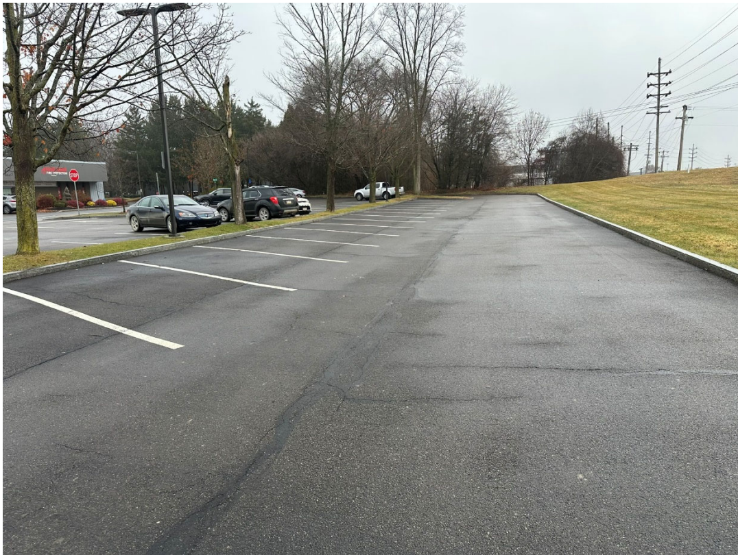
Photograph 2: City-Owned Parking Lot during November 2024 inspection (looking west).
