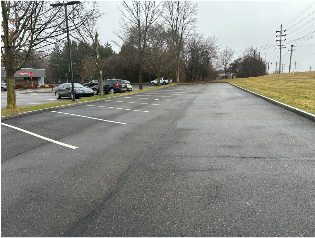
Photograph 1: City-Owned Parking Lot during November 2024 inspection (looking east).
