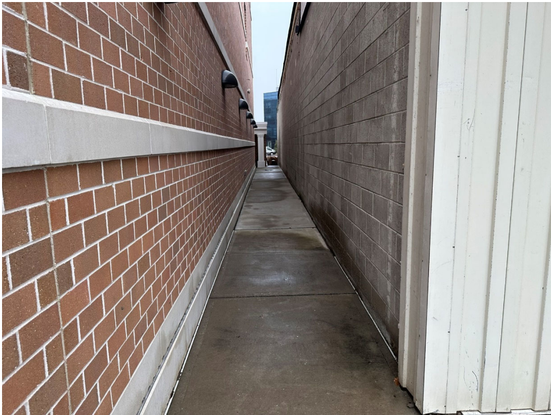
Photograph 6: Concrete cover system along east side of building (looking north).
