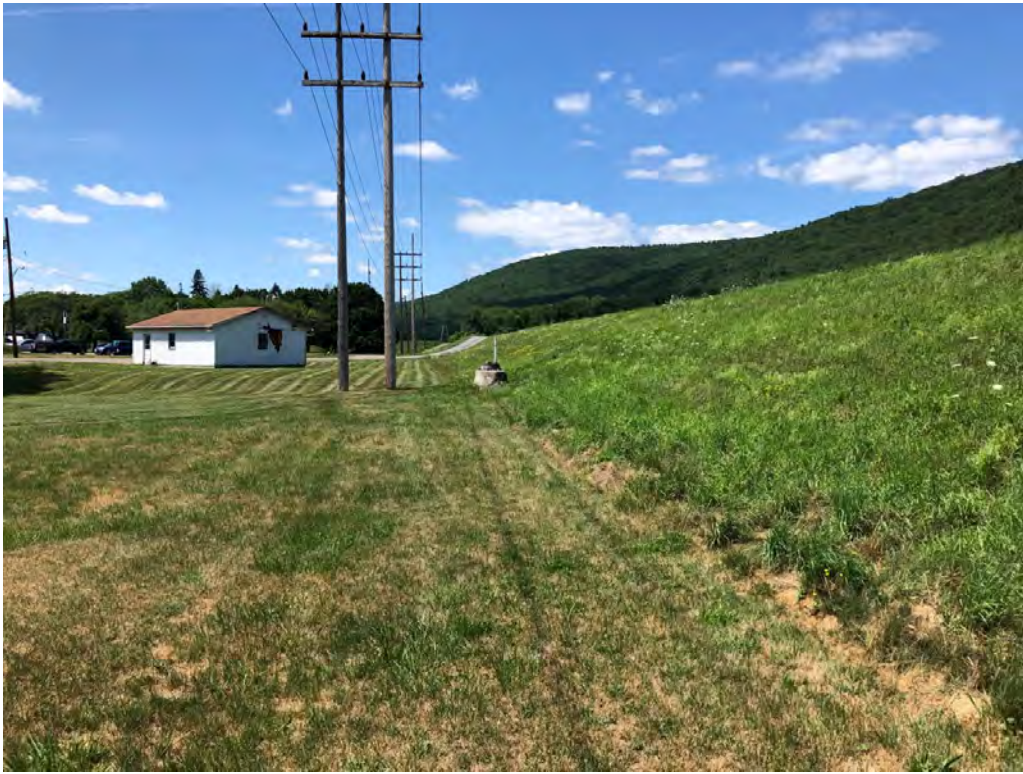
Looking northwest along the flood control berm, toward the garage building on Conhocton Street.
