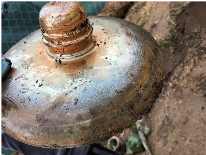
Picture 21: Opalescent insulator with approximately 1-ft diameter.
