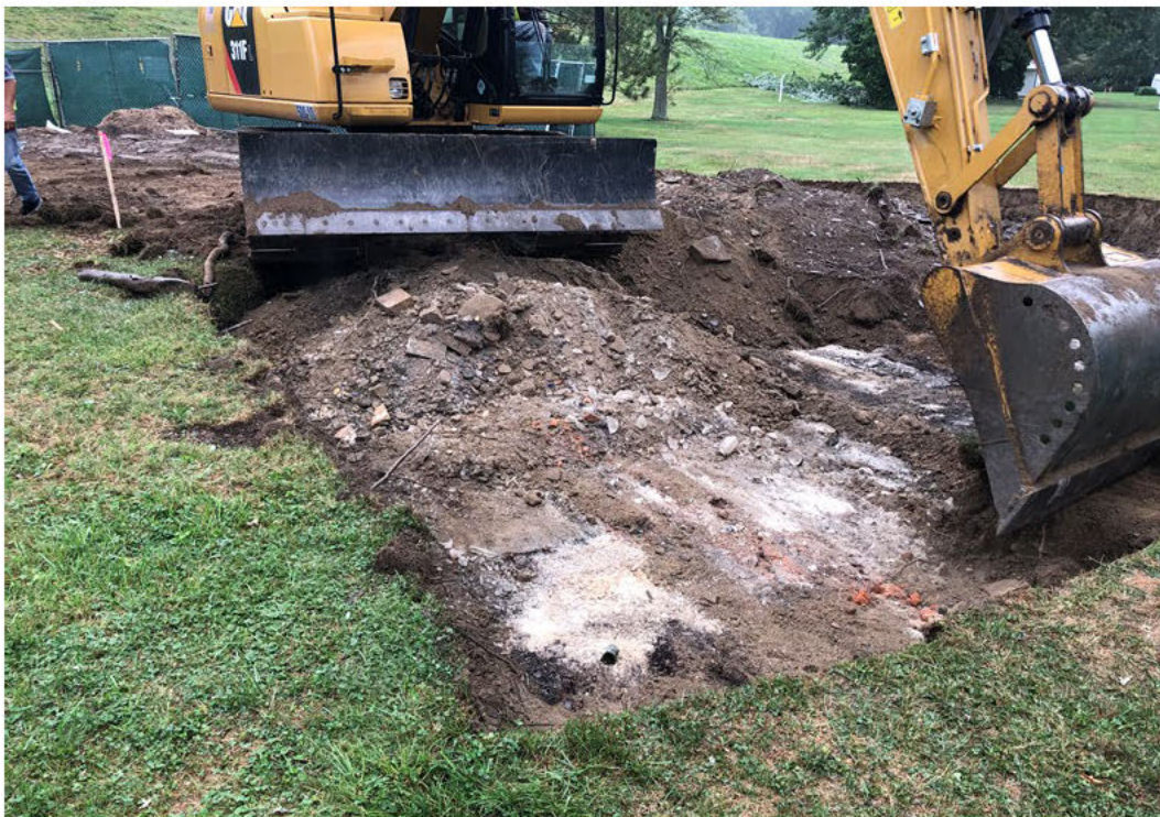
Picture 2: Excavation heavily impacted with ABG.
