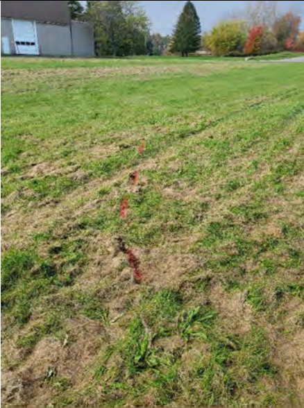
Photo 1: View of the subsurface obstructions marked out by Greencastle; assumed to be large field stones left within the swale embankment area near B412-OW-D's future location.
