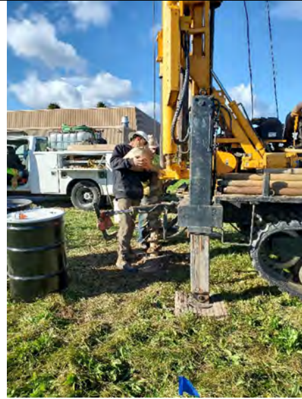
Photo 6: B412-OW-E receiving grout for casing stabilization.
