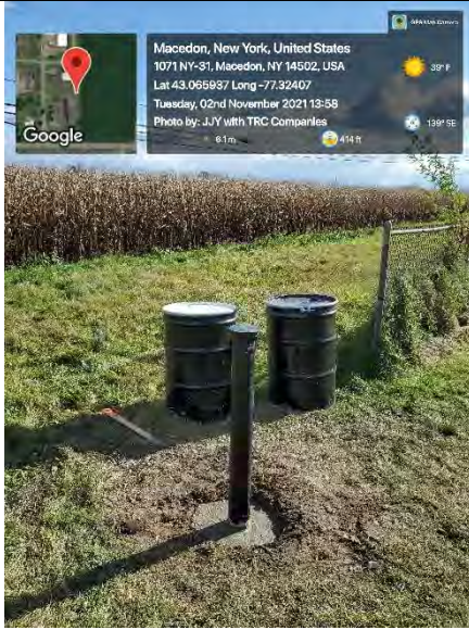
Photo 1: Final vicinity shot of B412-OW-E and its staged drums of soil excavation; grouted in place.
