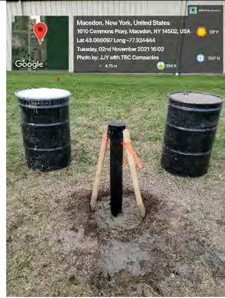
Photo 2: Final vicinity shot of B412-OW-D and its staged drums of soil excavation; grouted in place.
