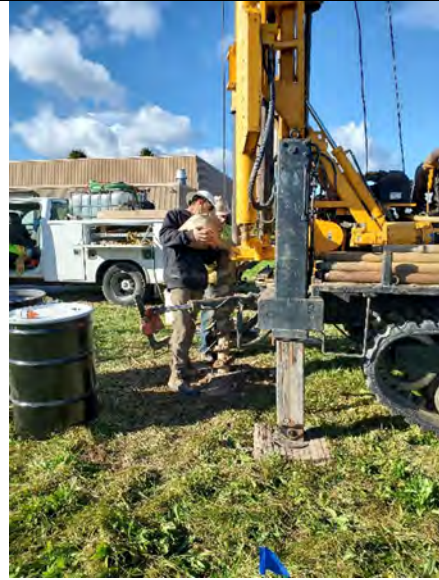
Photo 6: B412-OW-E receiving grout for casing stabilization.
