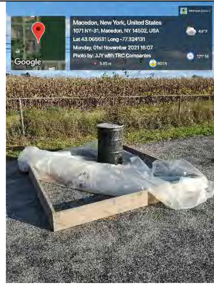
Photo 2: Decon station for LaBella PC within the Facility's parking lot; rolled up to prevent debris blowout from the previous days waste.
