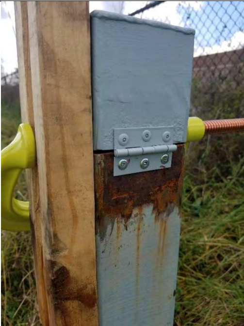
Photo 5: B103-OW-A's new cap and hinge; as fabricated by LaBella.
