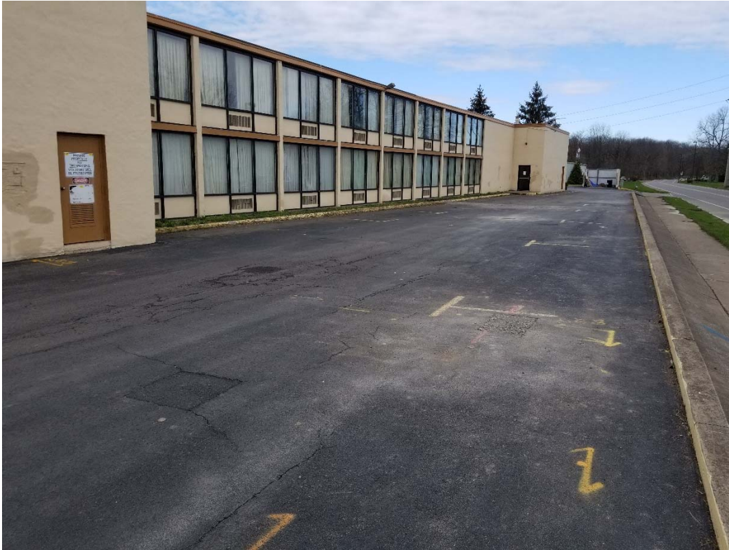
Photograph No. 1 – General view of building façade (north facing).
