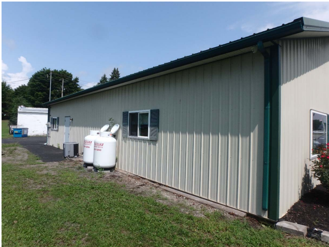
Photograph No. 2 – General view of building's western exterior wall.
