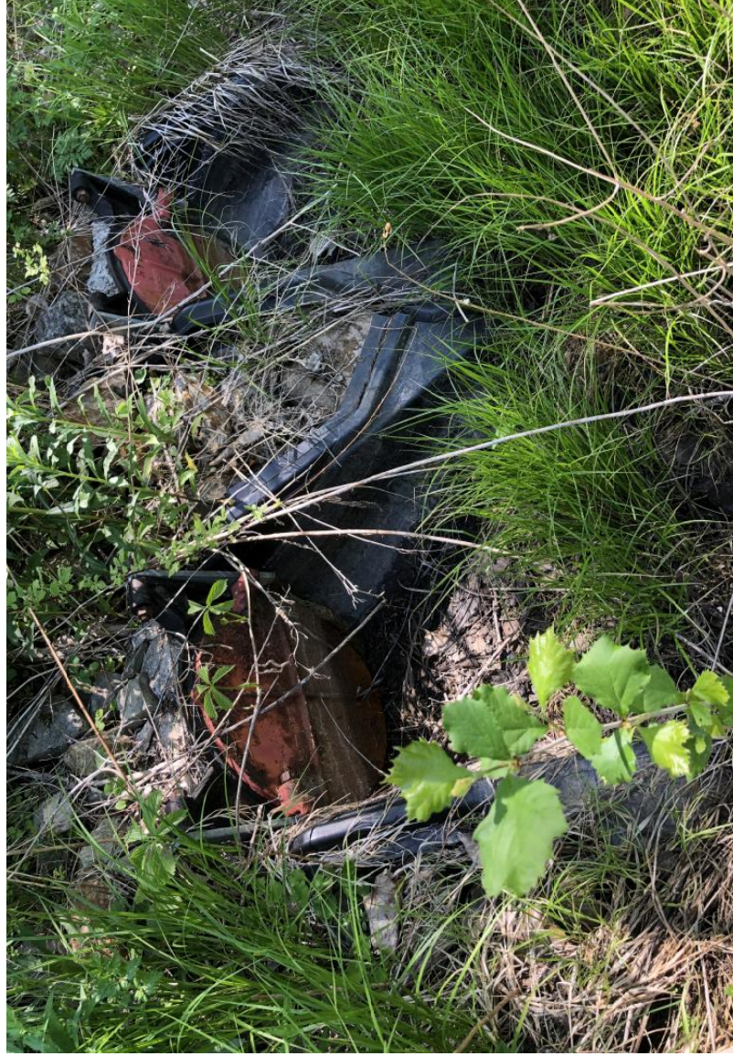
Photo #1: Outlet of West Disposal Area Drainage, looking north at flap gates.
