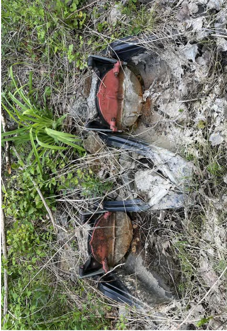
Photo #1: Outlet of West Disposal Area Drainage, looking north at flap gates.
