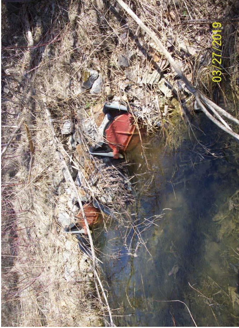
Photo #1: Flap gates, looking northwest.
