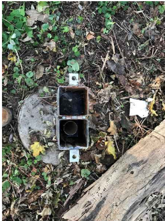
MW-4D – Well plug is missing.
