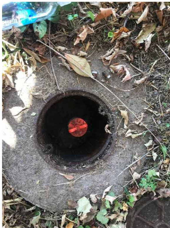
MW-6 – Well head in good condition.
