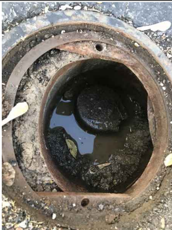
MW-5 – Well head cap cannot be removed.
