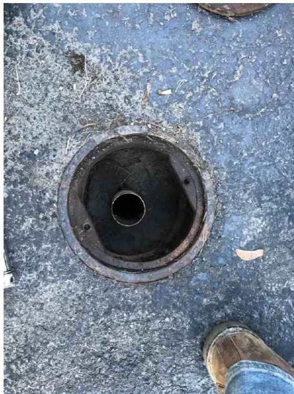
MW-2S –Well plug is missing.
