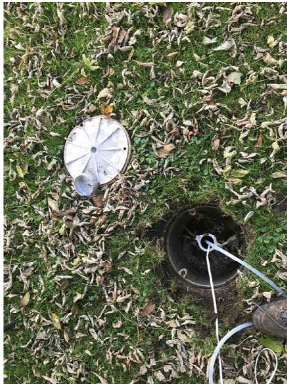
MW-3A – Inner well cap is damaged but functional.
