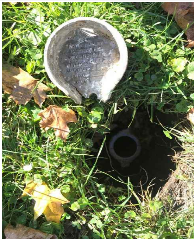
MW-1 – Inner well cap is damaged but functional.
