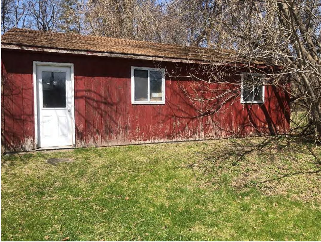
South side of NYSEG garage structure - viewing north
