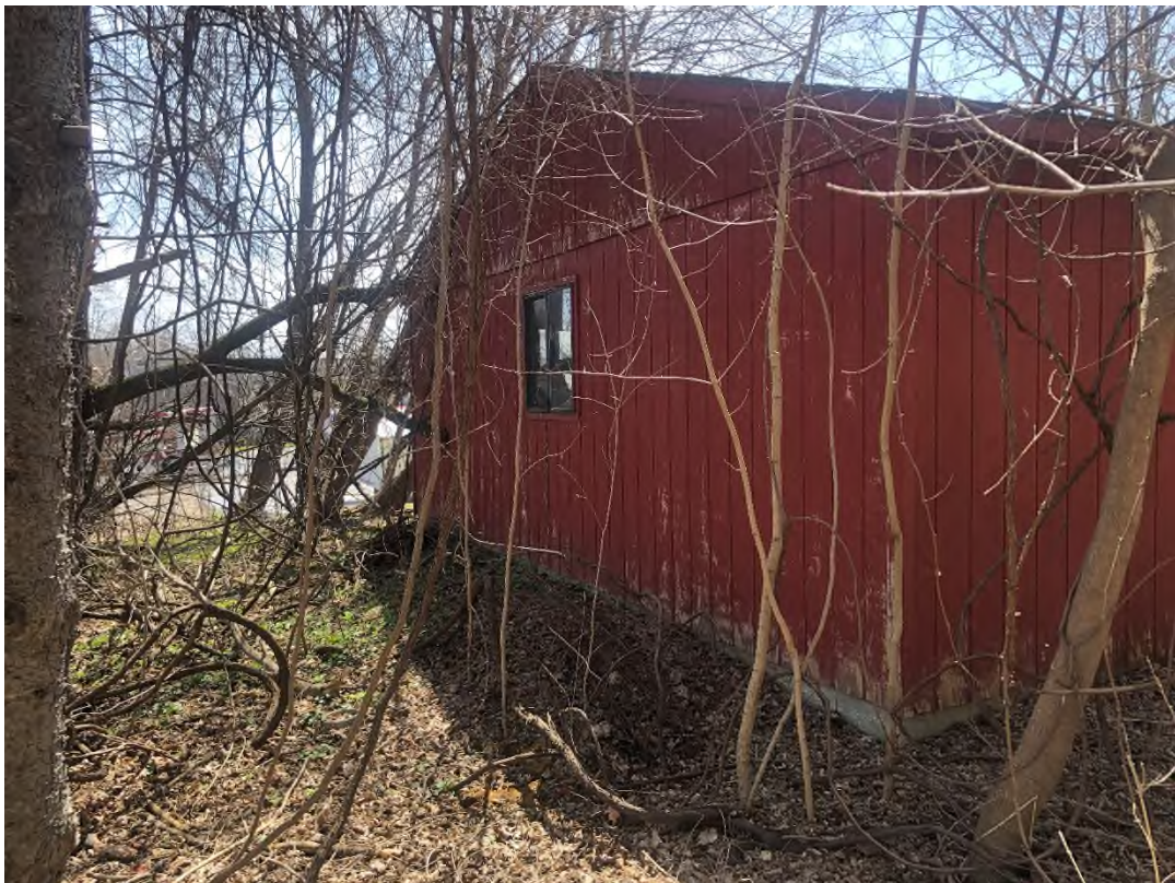
Back (east) side of NYSEG garage structure - viewing southwest
