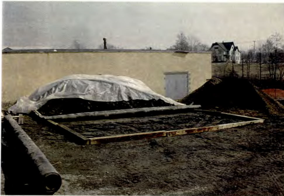
HIGH DENSITY POLYETHYLENE LINED HOLDING AREA
