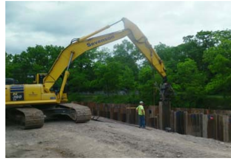
Installation of bank area structural sheets after splice
