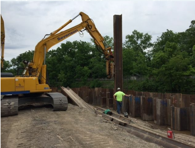
Threading 22' structural sheeting along south side of the historic structure.
