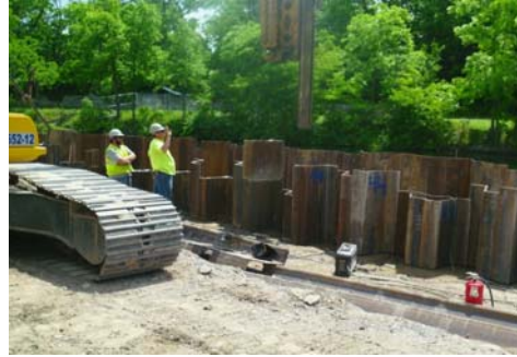
SES crew preparing to thread a top section of AZ-48 sheet pile to be spliced and driven to final depth
