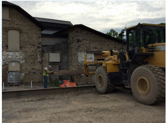
Prepping sheetpile for welding procedures.
