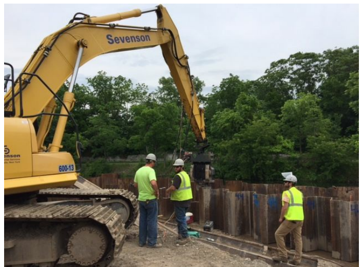
Excavator mounted variable moment hammer driving welded sheetpile to desired elevation.
