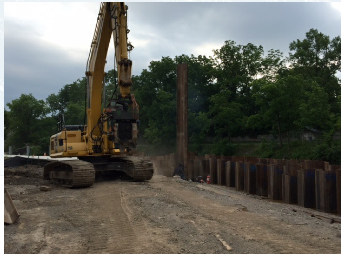
Positioning PC360 equipped with VM hammer to drive sheetpile following completion of welding procedures.
