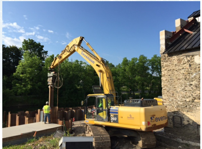
Driving welded 44' sheetpile with variable moment hammer.
