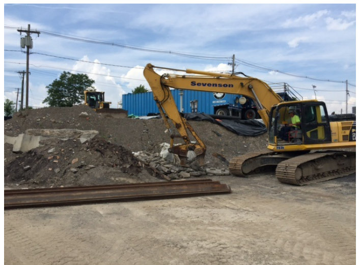
PC 220 with cruncher sizing concrete material for disposal.
