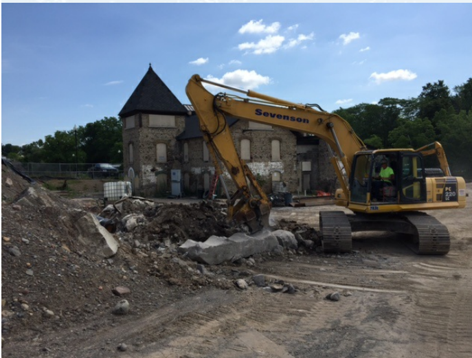
Continuing to size concrete debris for disposal.
