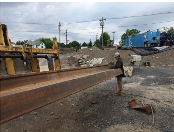
Cutting leads into locks of 22' sheetpile to ease with threading.
