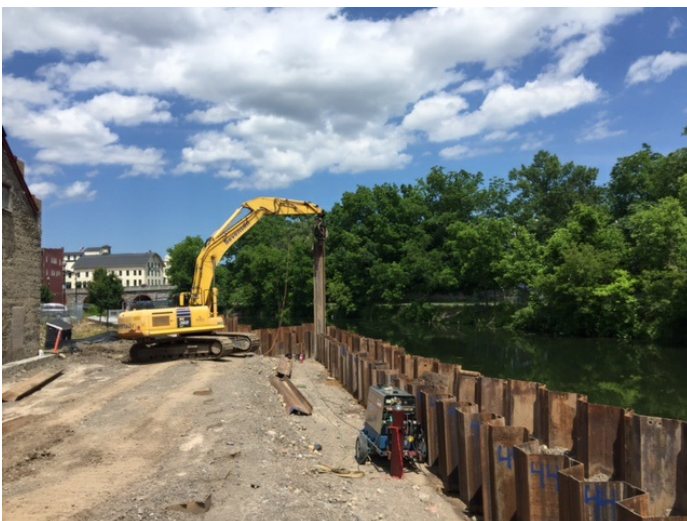
Utilizing excavator mounted variable moment hammer to drive welded sheetpile.
