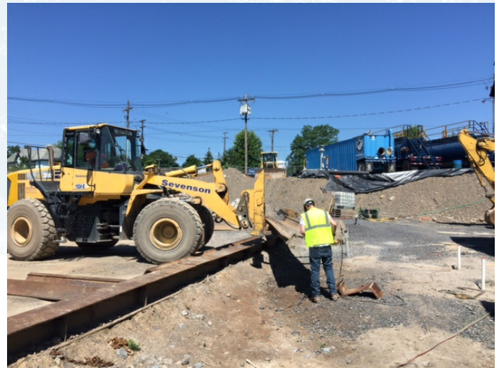
Prepping sheets for installation by grinding and beveling ends of sheets.
