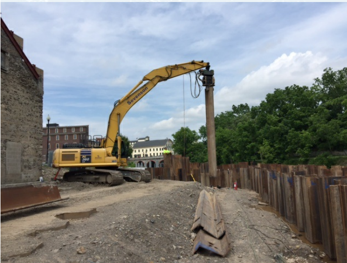
Utilizing excavator mounted VM hammer to drive welded sheetpile to desired elevation.
