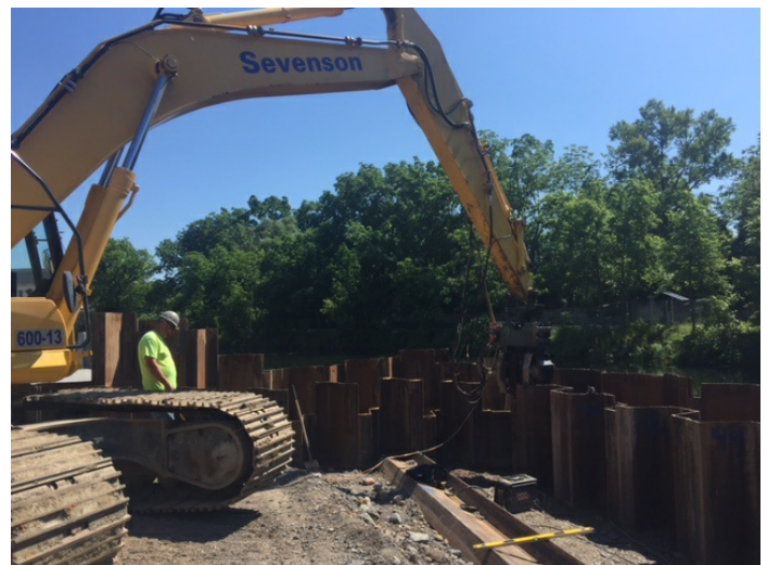
Driving sheetpile to desired elevation along south side of the historic structure.
