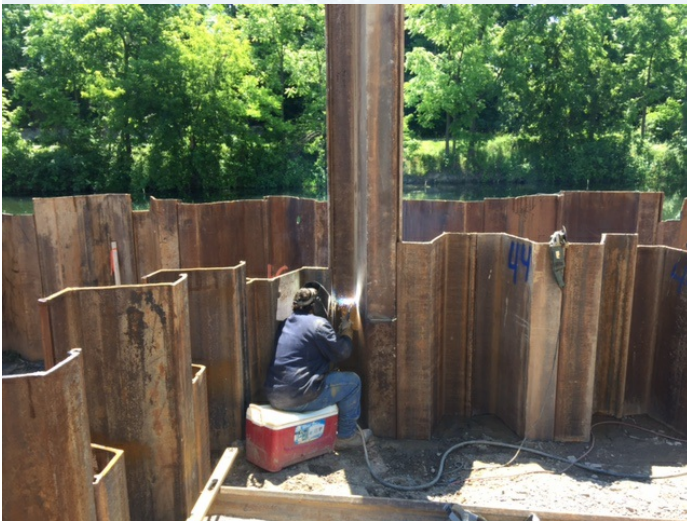
Continuing welding procedures on the structural sheeting.
