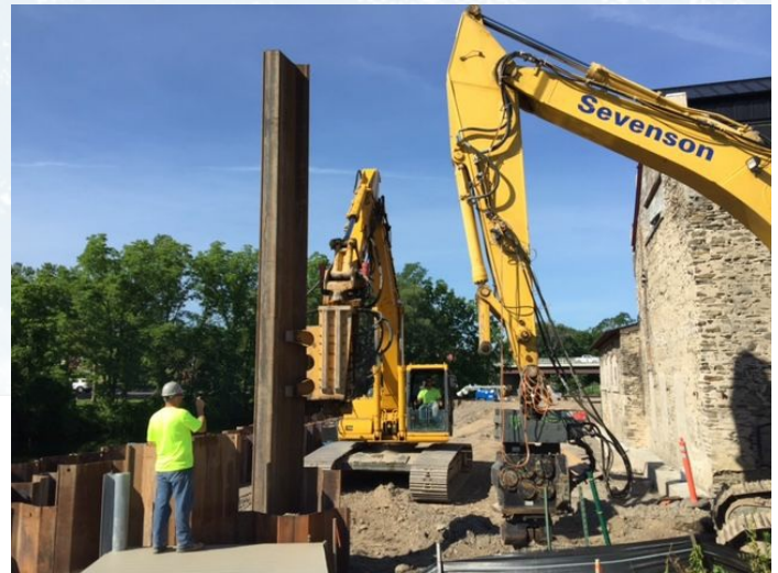
Threading sheetpile utilizing PC220 with Robovibe attachment.
