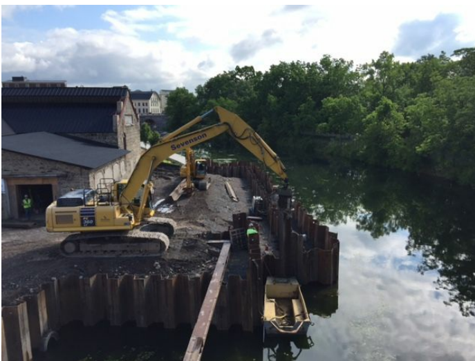
Completing west side of the structural sheetpile installation utilizing excavator mounted variable moment hammer.
