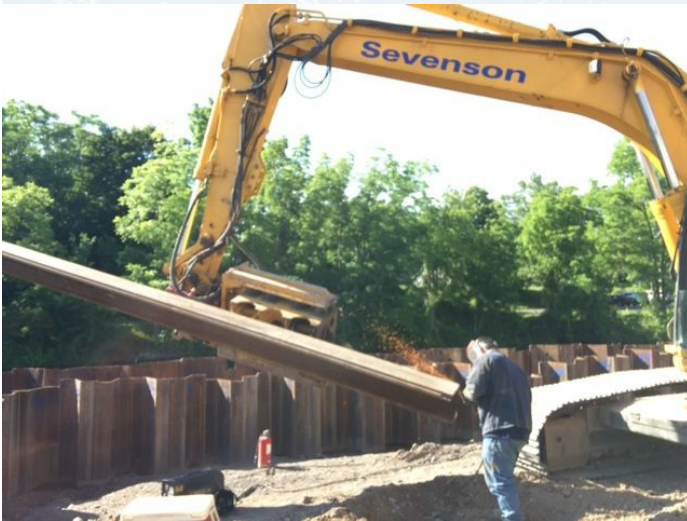
Grinding 22' sheetpile prior to welding procedures.
