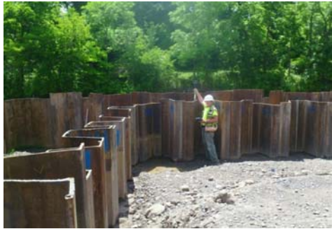
Thew surveying structural sheet tops
