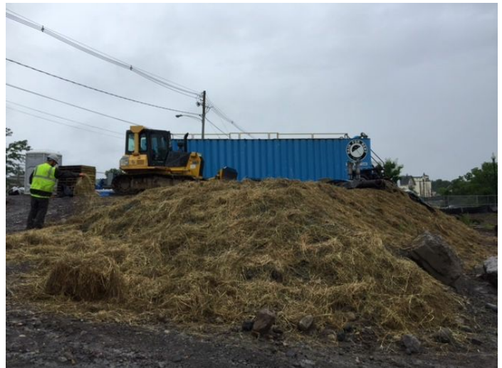
Placing grass seed and hay for additional means of erosion control prior to shutdown.
