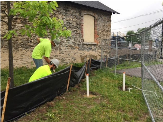
Reinstalling silt fence along west side of the historic structure.
