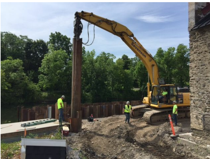
Driving welded sheetpile to desired elevation.
