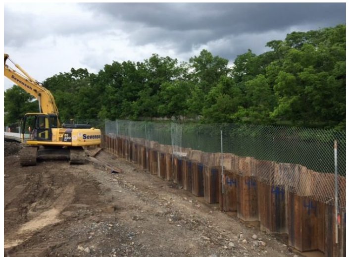
Sevenson installed additional site security fence along the top of the structural sheetpile prior to shutdown.
