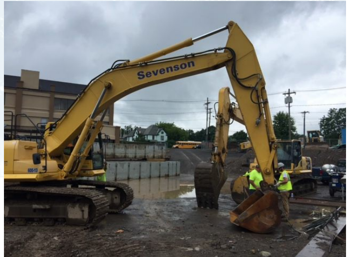
Following completion of structural sheetpile installation, reattaching bucket to PC360 prior to demobilization.
