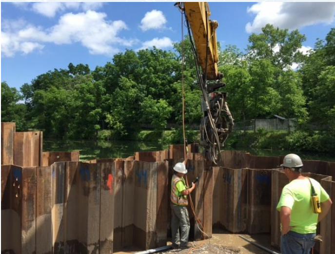
Surveyor on-site to check elevations of driven structural sheetpile.
