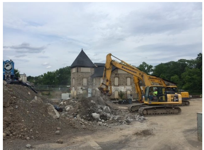
Sizing concrete debris for disposal.
