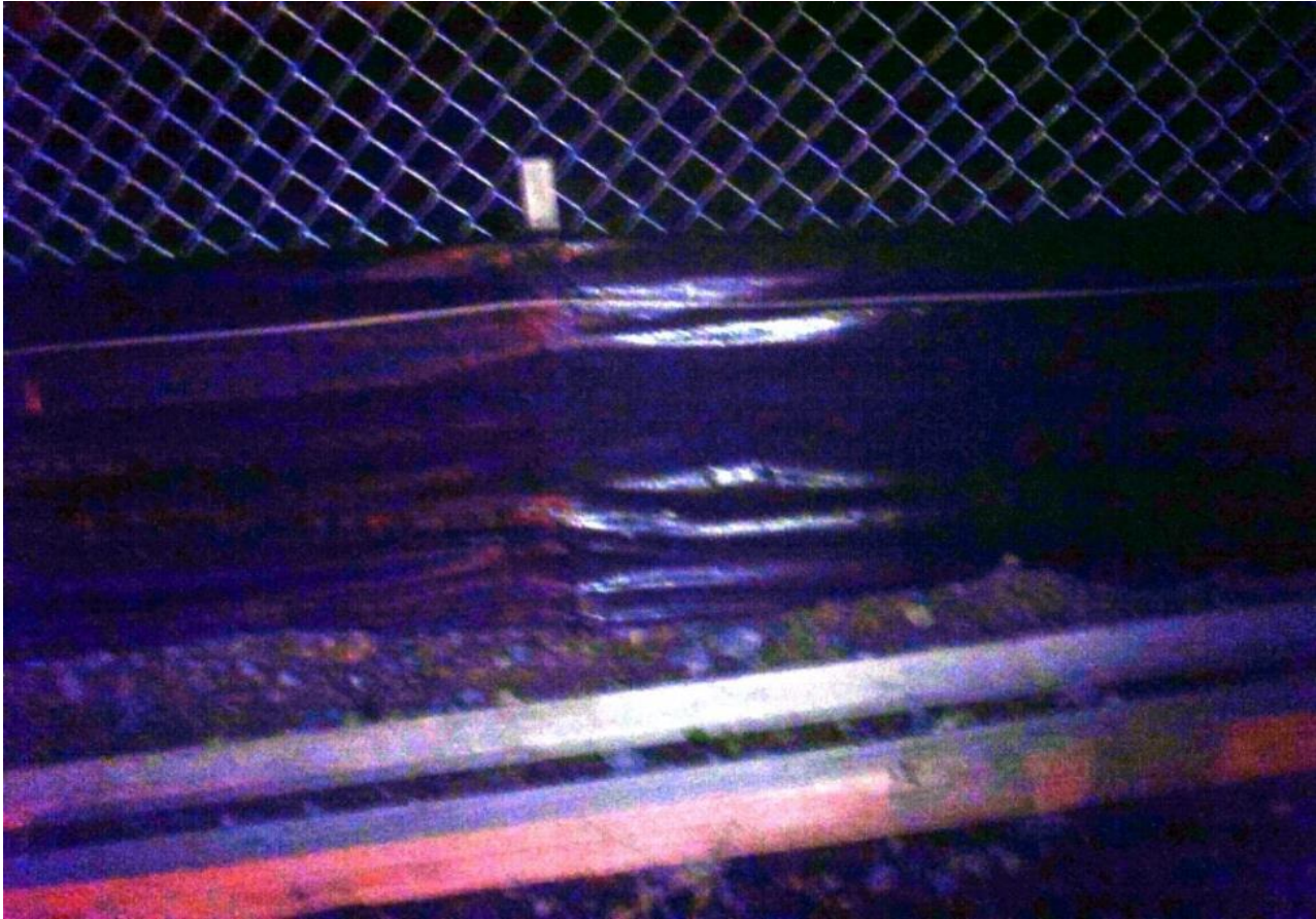
Silt fence along west side of site repaired
