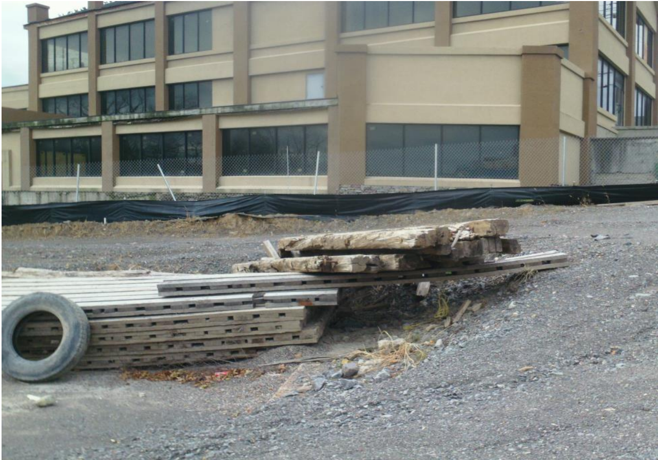
Silt fence along west side of site
