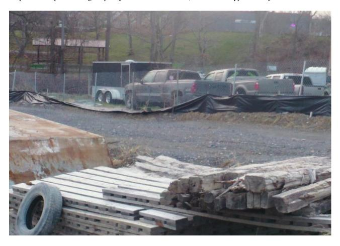
Silt fence along west side of site collapsed.
