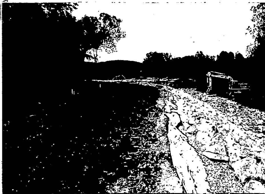
WEST DIKE STATION 14+00 PLACEMENT OF RIPRAP, BEDDING AND GEOTEXTILE FABRIC
