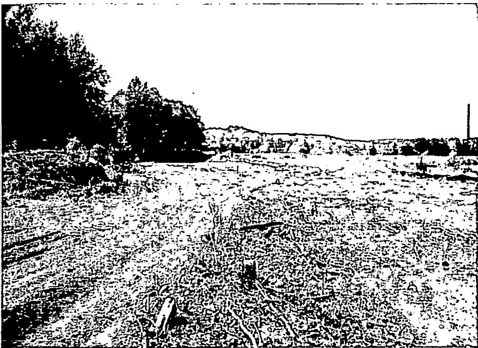
DIKE FOUNDATION CLEARING WEST DIKE 9+00
