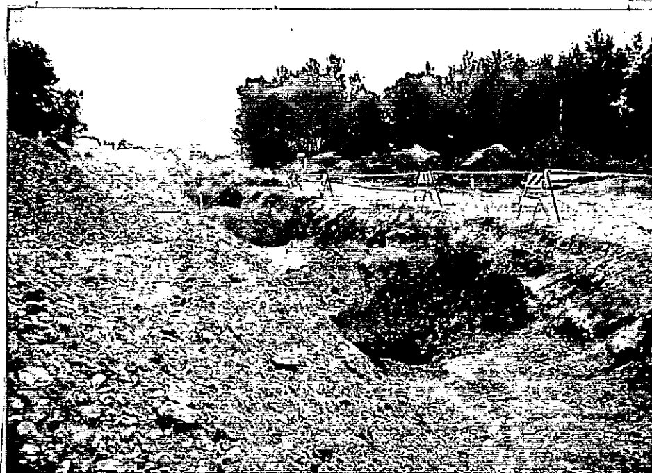
KEY TRENCH EXCAVATION WEST DIKE STATION 4+50 TO STATION 7+50
