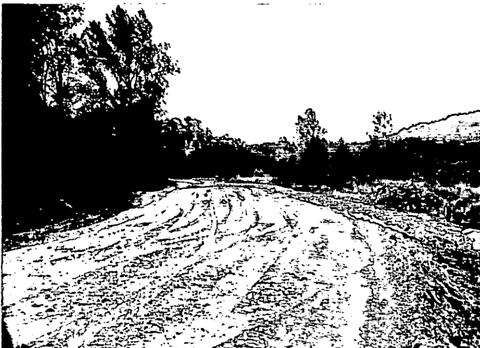
TOE TRENCH WEST DIKE STATION 16+50
