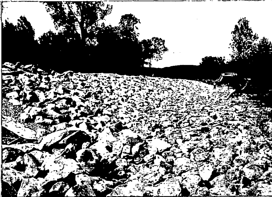
WEST DIKE STATION 13+50 PLACEMENT OF RIPRAP
