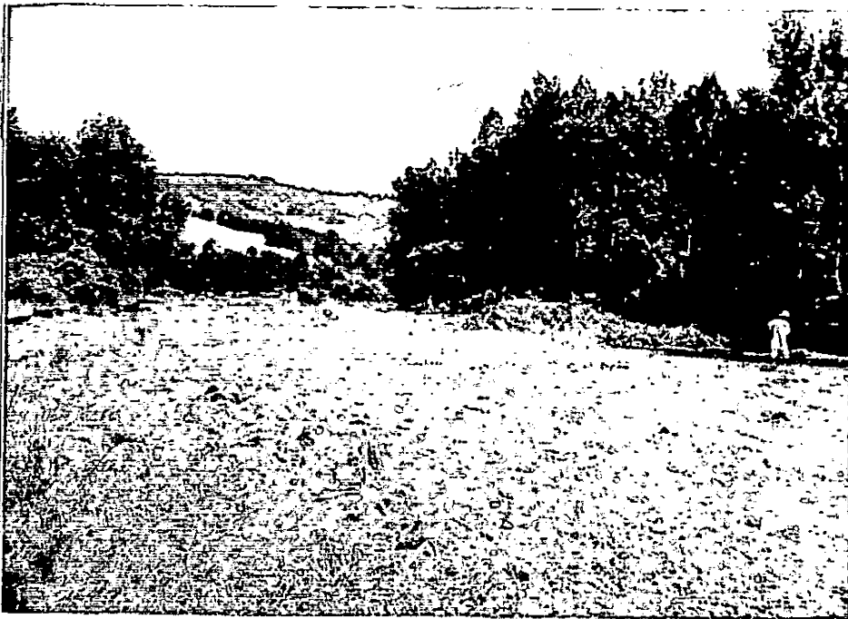
DIKE FOUNDATION CLEARING WEST DIKE STATION 6+00
