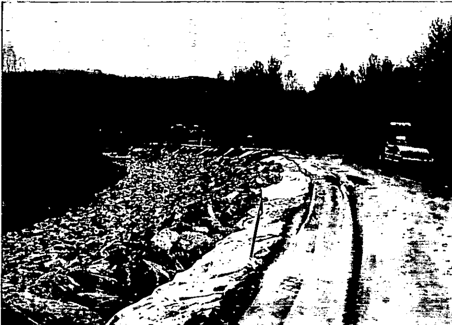
WEST DIKE STATION 1+50 PLACEMENT OF RIPRAP
