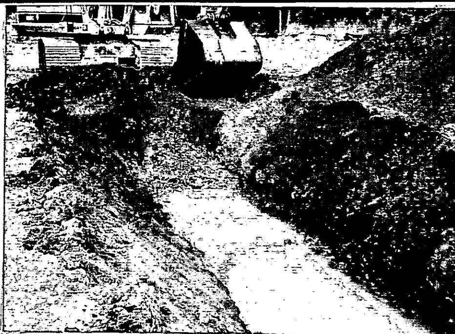
KEY TRENCH EXCAVATION WEST DIKE STATION 16+00
