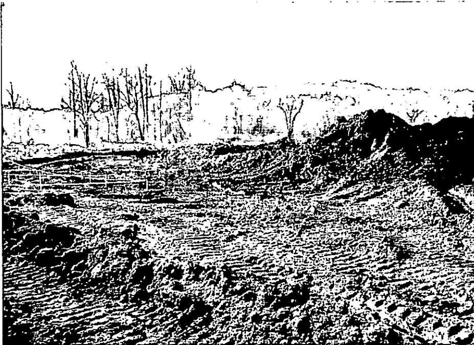
SOUTH LANDFILL AREA EXCAVATION
