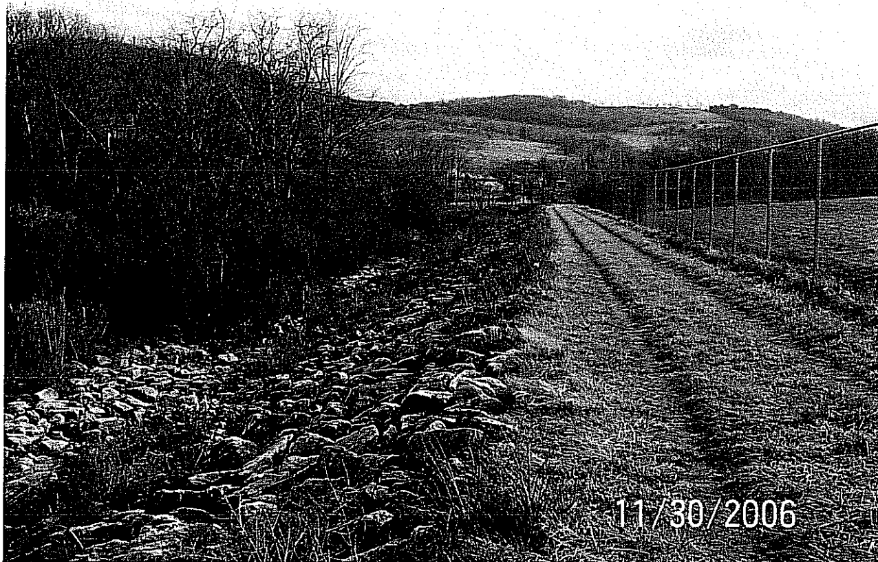
11/30/2006 West Dike Station 6+00 view to the South
