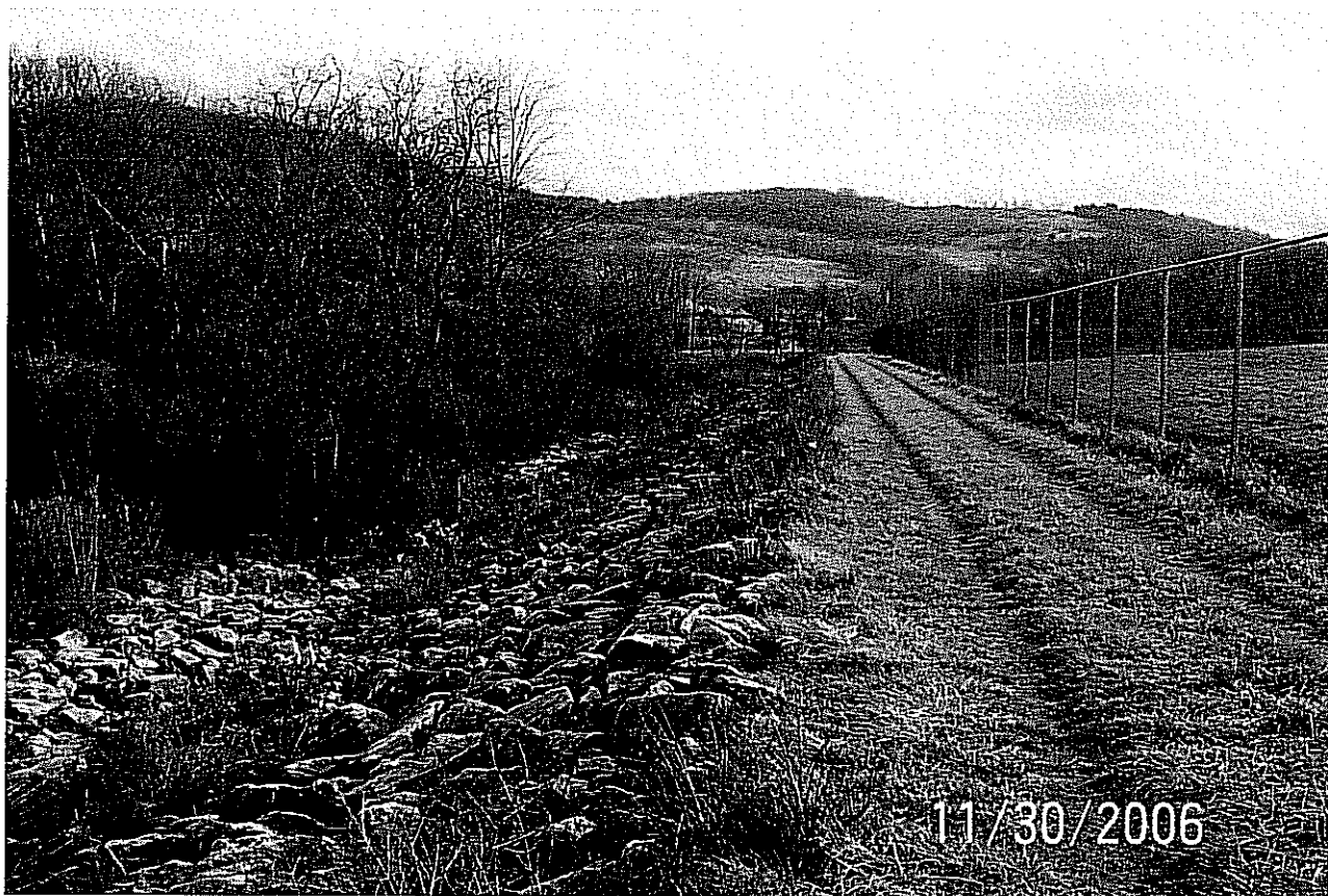
11/30/2006 West dike station 24+00 view to the North
