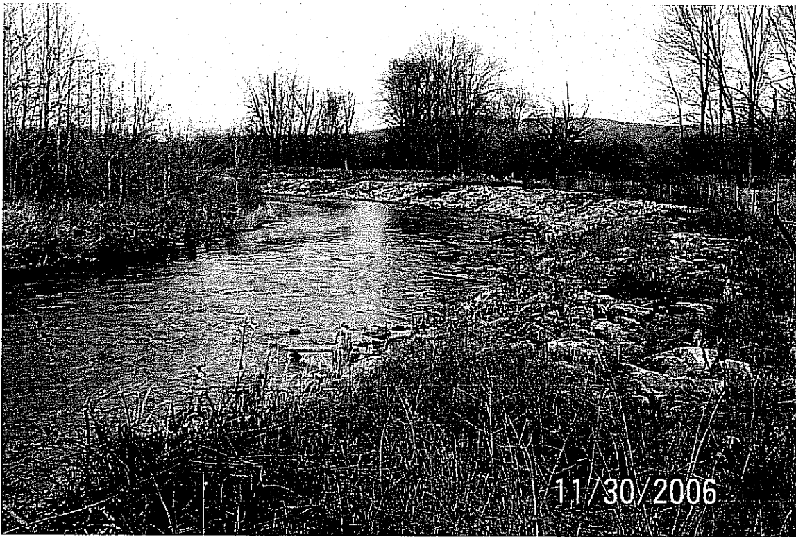
11/30/2006 East Dike Station 17+00 view to the North
