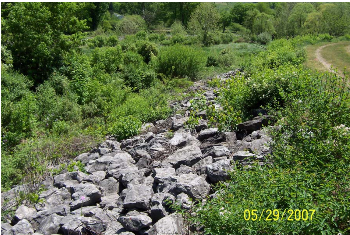
5/29/2007 West Dike Station 10+00 view to the South
