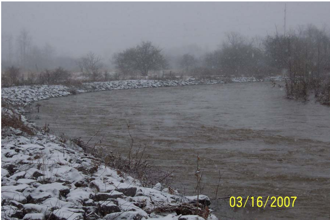
3/16/2007 East Dike Station 16+00 view to the South
