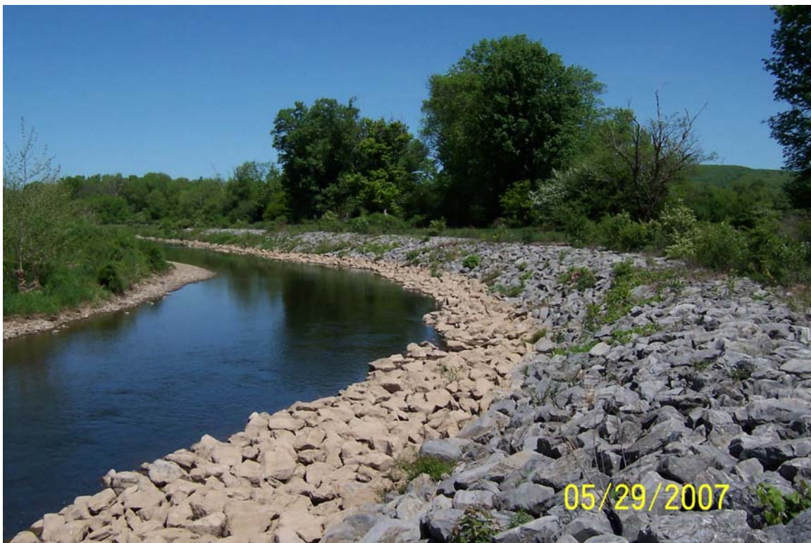
5/29/2007 East Dike Station 18+00 view to the North
