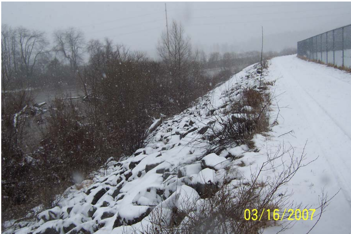
3/16/2007 West Dike Station 16+00 view to the South
