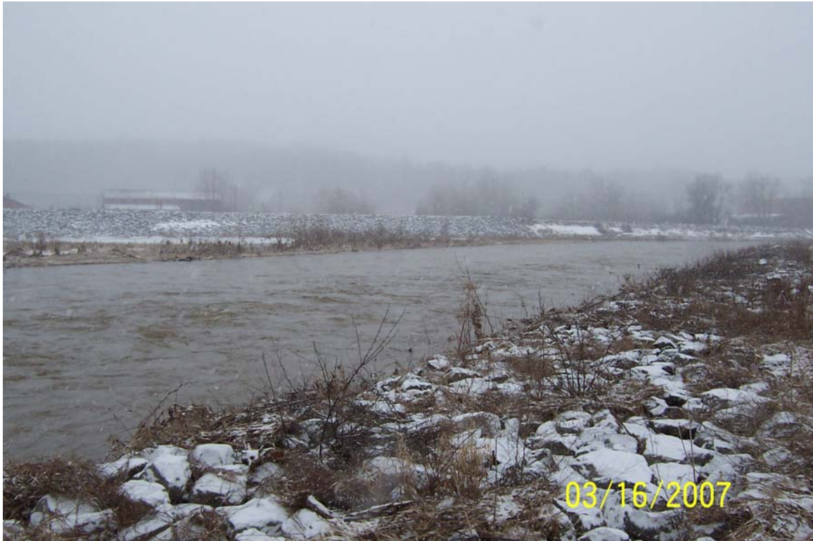
3/16/2007 East Dike Station 4+00 view to the North
