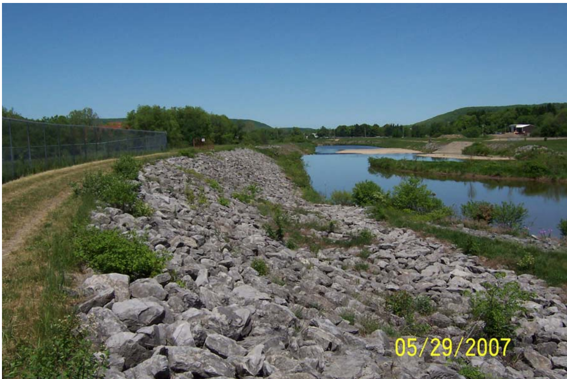
5/29/2007 West Dike Station 4+00 view to the North
