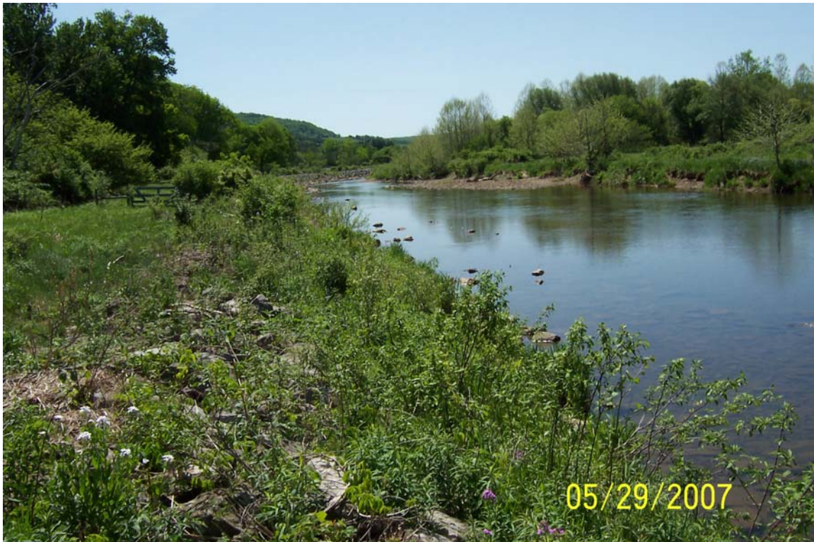
5/29/2007 East Dike Station 8+00 view to the South
