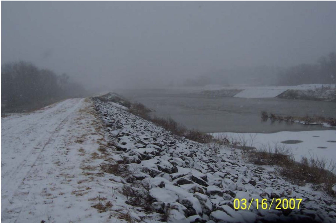
3/16/2007 West Dike Station 2+00 view to the North
