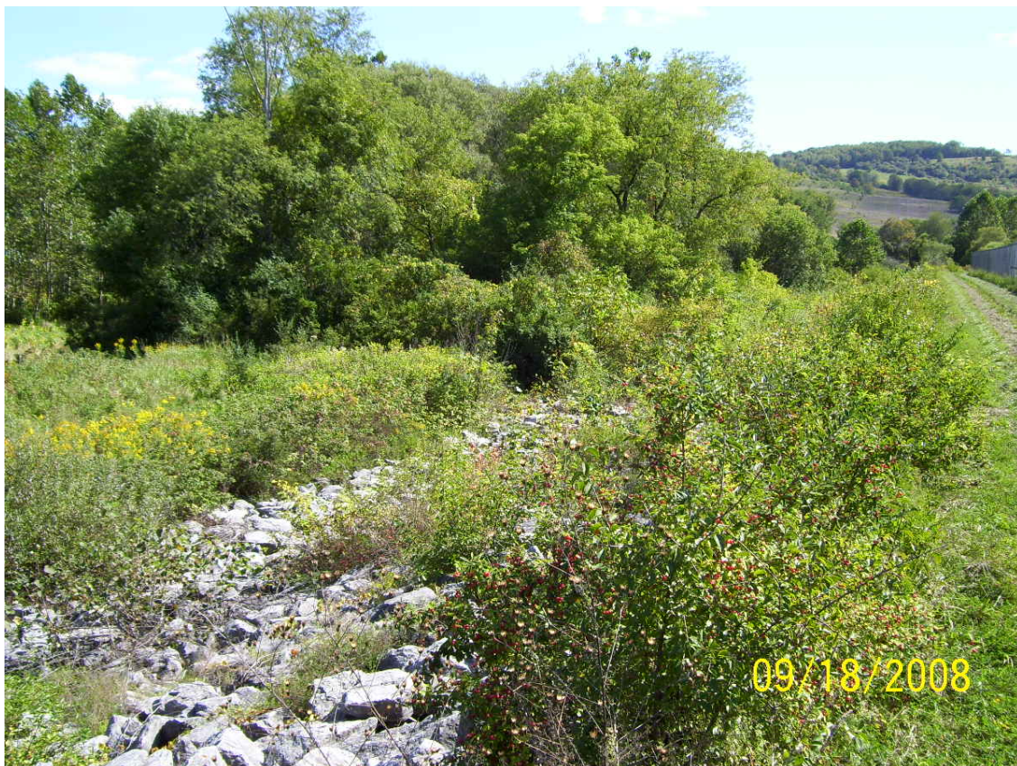
Annual low flow inspection – West dike station 6+00 view to the South
