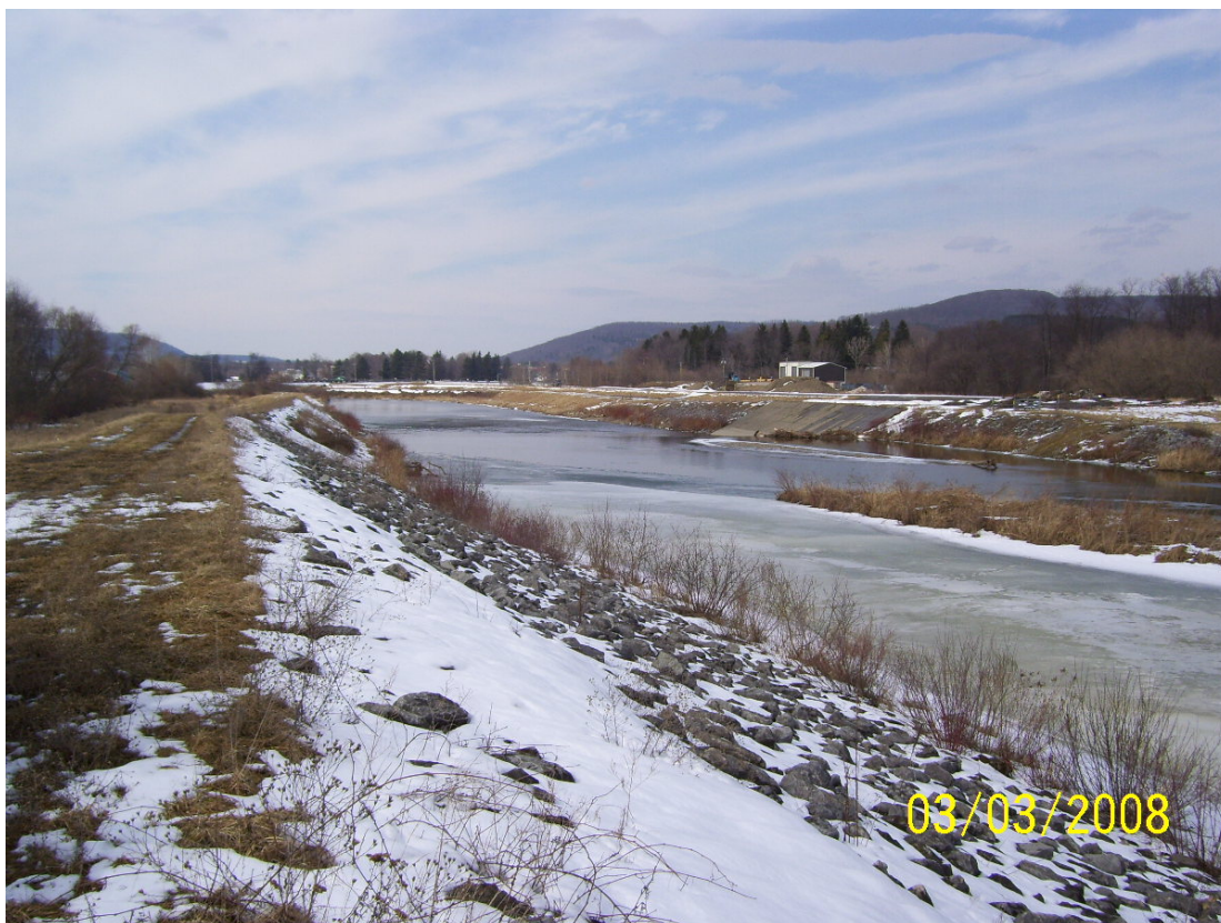
Post high water – West dike station 2+00 view to the North
