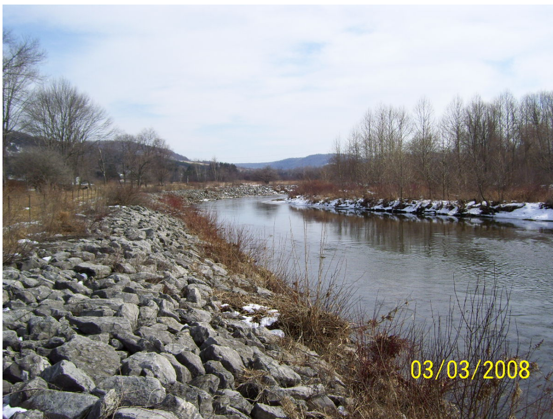
Post high water – East dike station 12+00 view to the South
