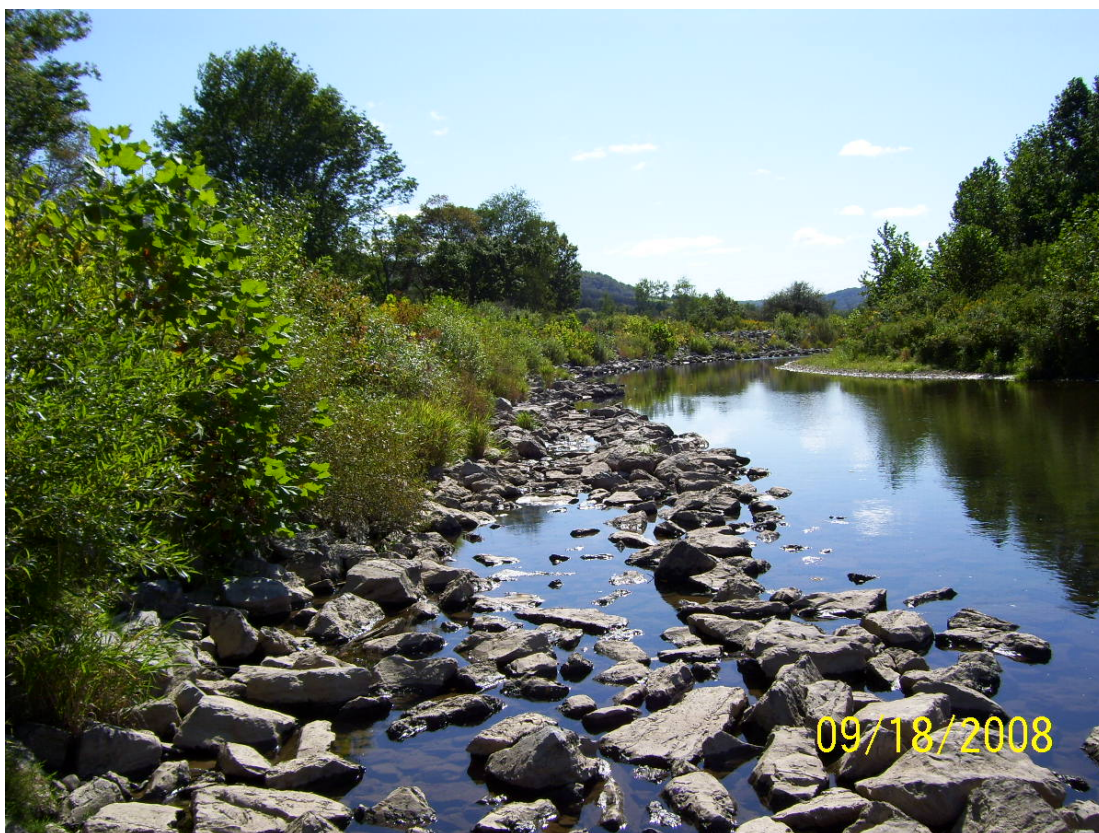
Annual low flow inspection – East dike station 12+00 view to the South
