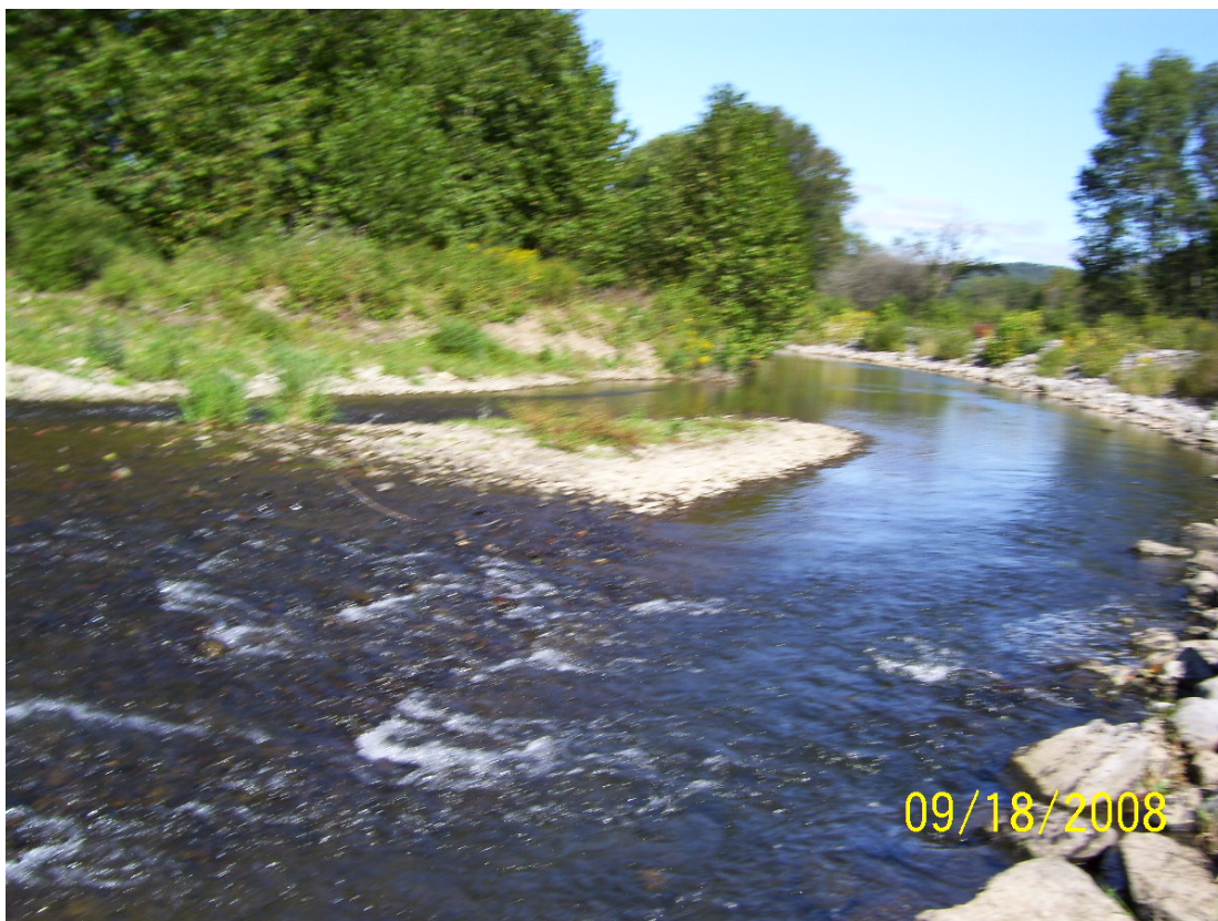
Annual low flow inspection – East dike station 18+00 view to the North
