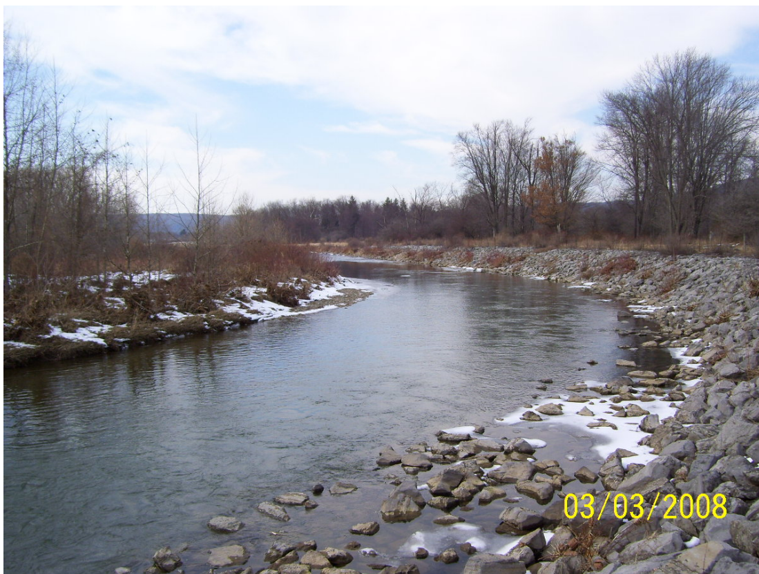
Post high water – East dike station 18+00 view to the North
