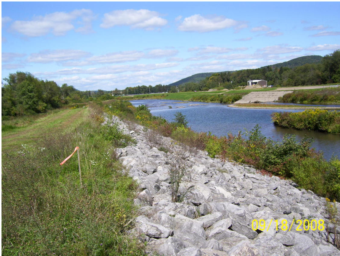
Annual low flow inspection – West dike station 2+00 view to the North
