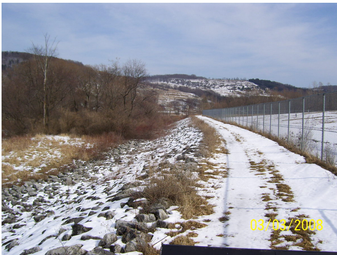
Post high water – West dike station 6+00 view to the South
