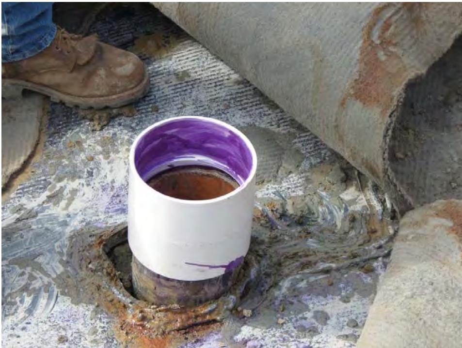
10/17/12: Replaced gas vent V-12 coupling
