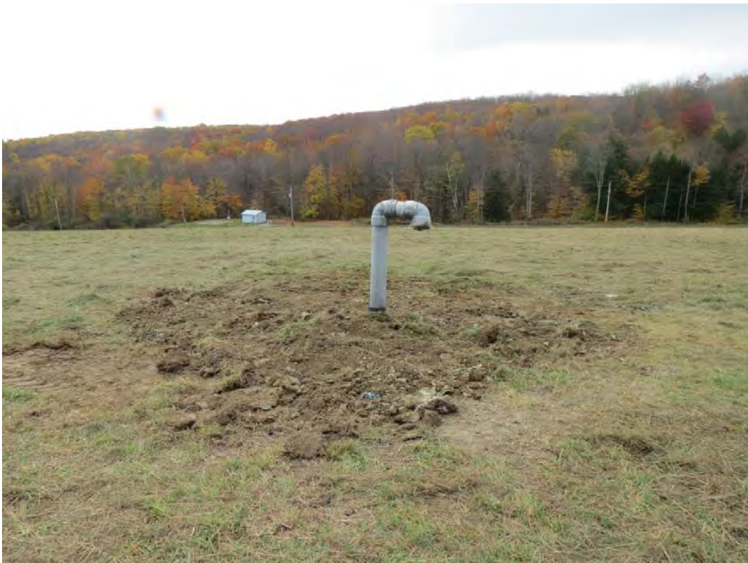
10/17/12: Gas vent V-12 repairs complete
