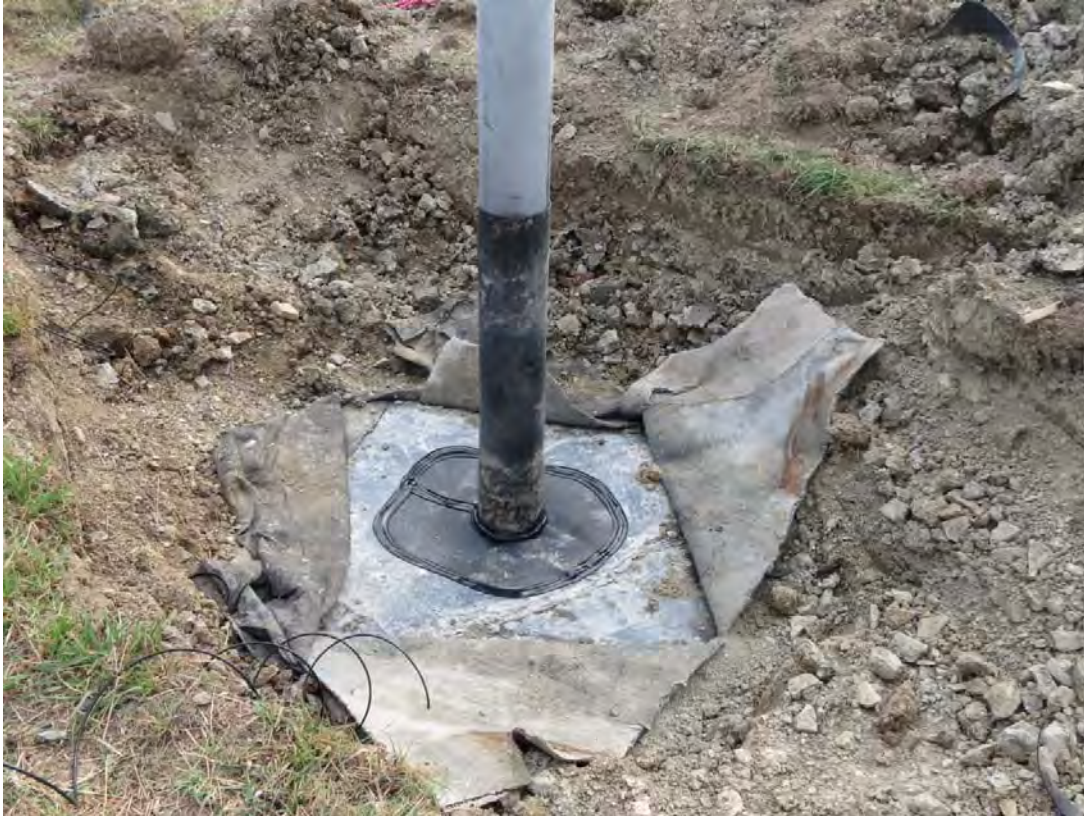
10/17/12: Liner repair complete at gas vent V-12
