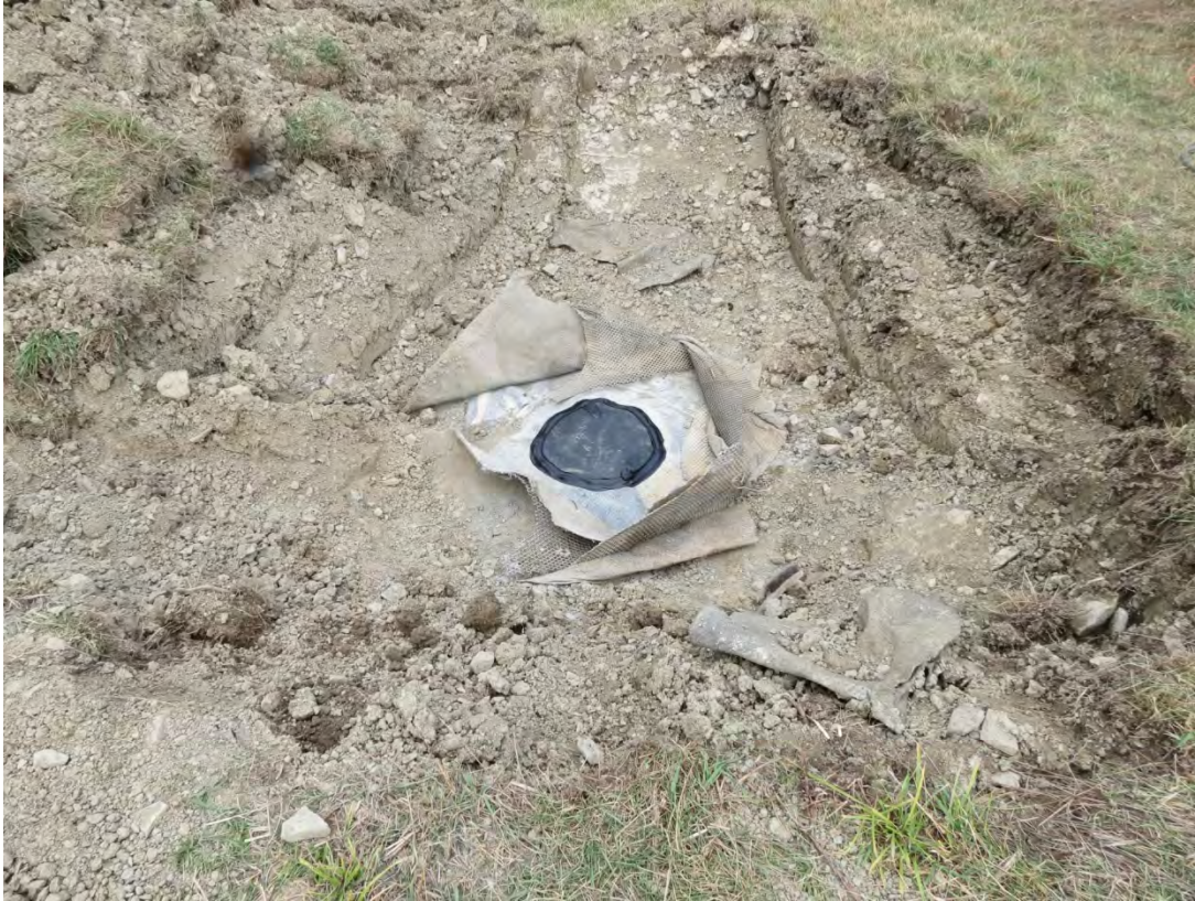
10/17/12: Completed liner patch at PZ-3R location
