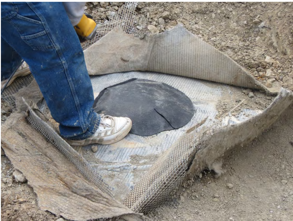
10/17/12: Liner repair in progress at PZ-3R location
