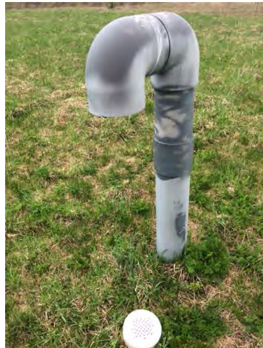
Photo No. 8 Landfill gas vent
