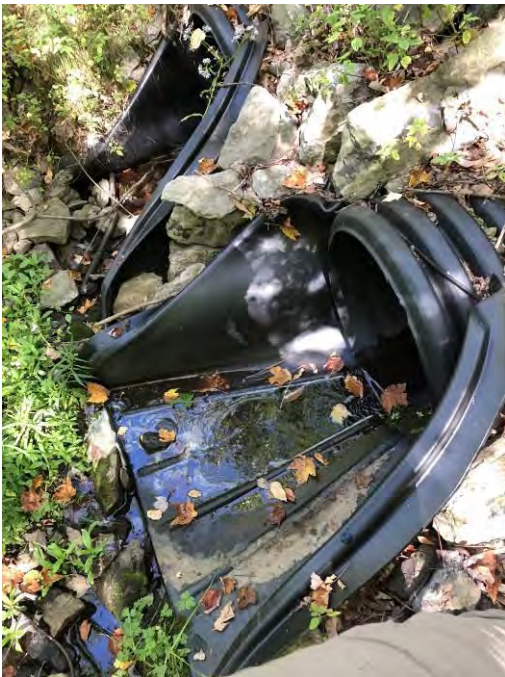
Photo No. 3 SW-2
