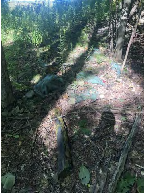
Photo No.5 Exposed geotextile
