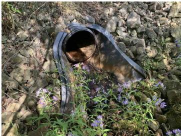
Photo No. 5 View of exposed geotextile by the access road to MW-04.
