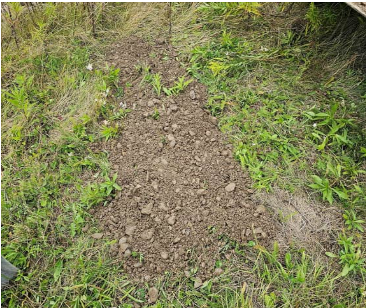
Photo No. 7 Typical Recovering of Geotextile above cap.
