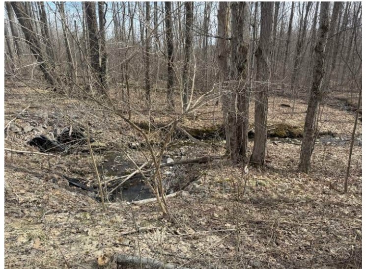
Photo No. 8 Access Road culverts west of SW-3.
