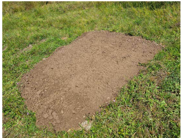
Photo No. 8 Typical Recovering of Geotextile above cap.
