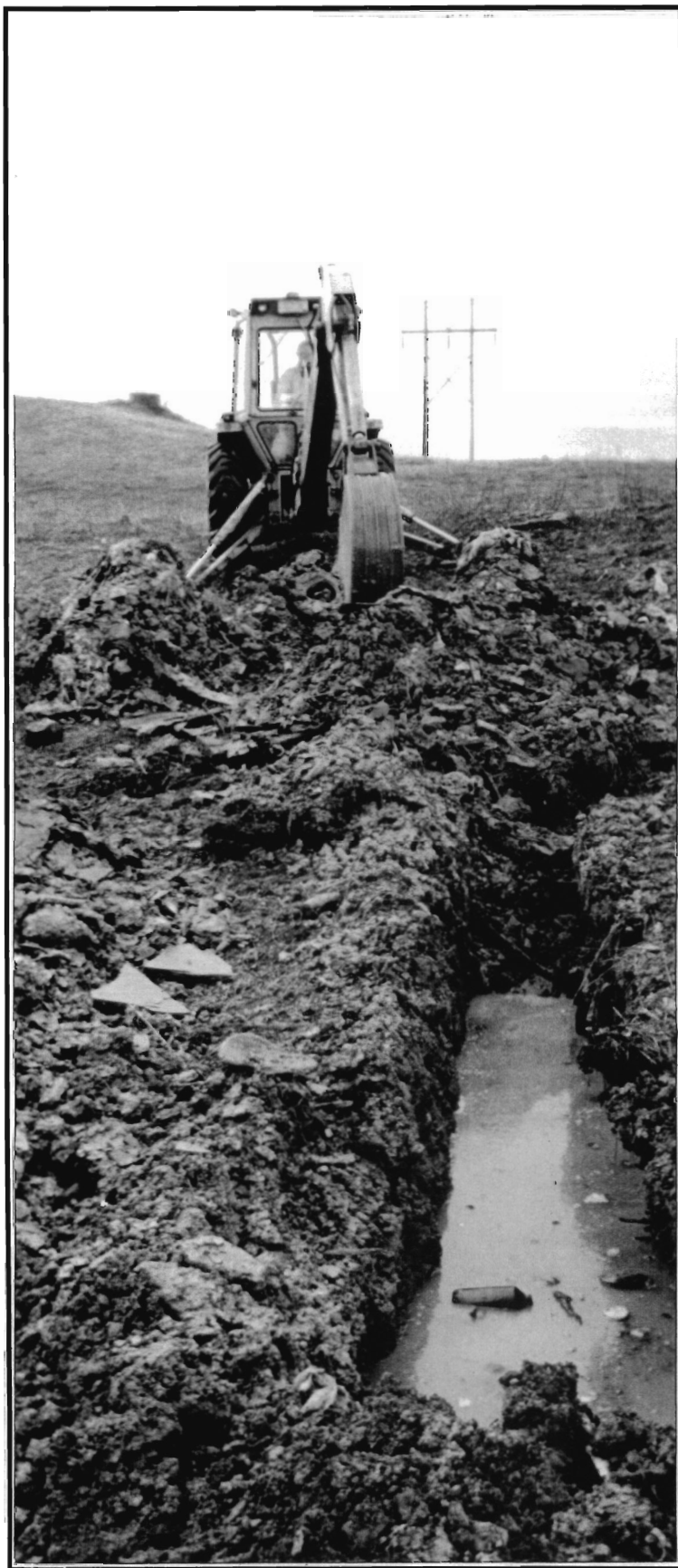
Test Pit Excavation - TP2 Uncovering Unreported Fill Between Busy Bee and Henry Landfills
