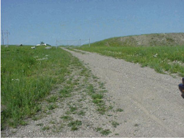
Access Road and Gate 6/15/01
