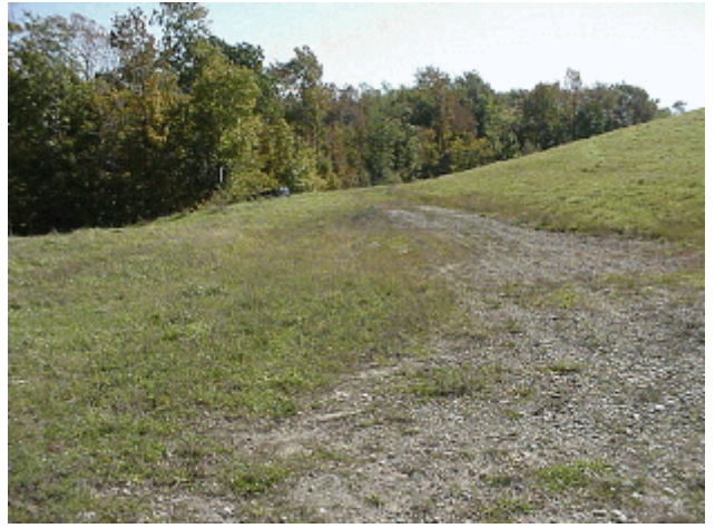
Northeast Corner Cap Area
