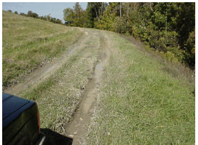
Northeast Corner Cap Area
