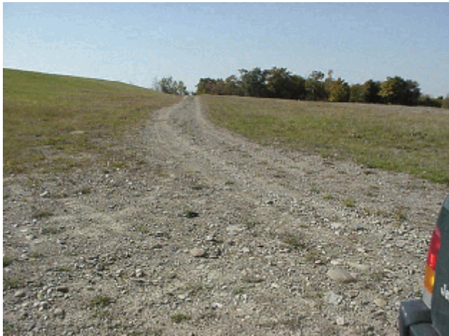
North side Cap Area/Perimeter Road
