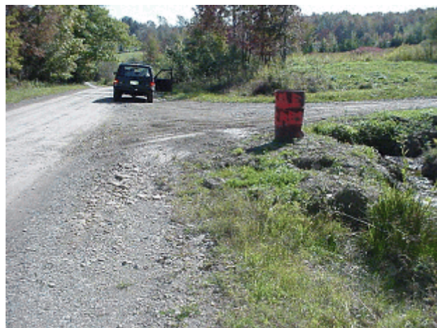
Clark Road entrance
