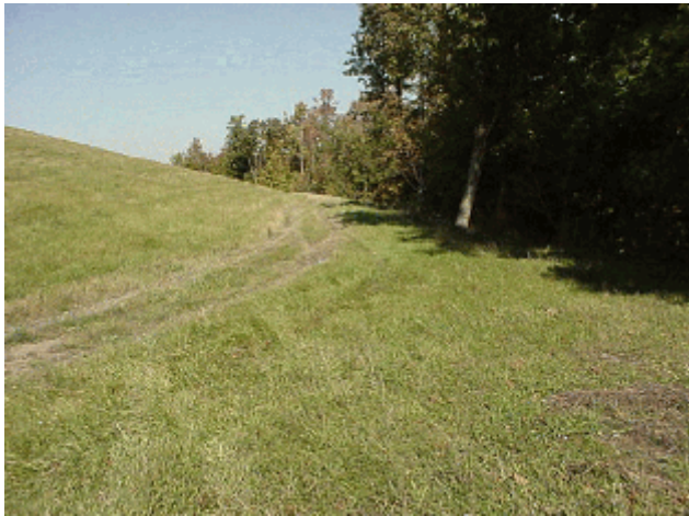
South East Corner Cap Area
