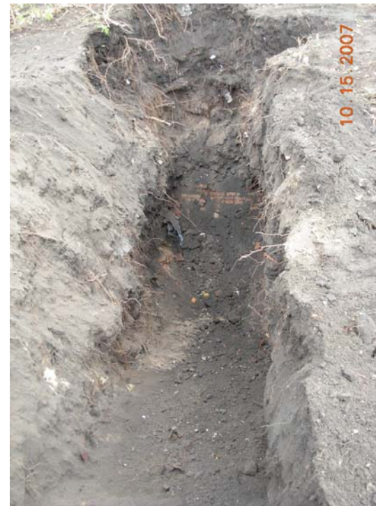
Test Pit 5 with the brick foundation ~12' bgs.
