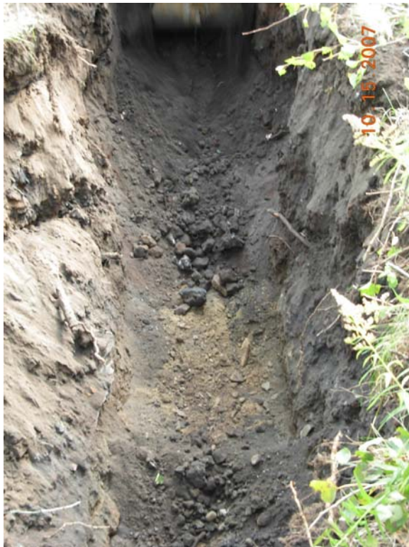
55-gallon drum encountered in Test Pit 6 (“green resin” material)
