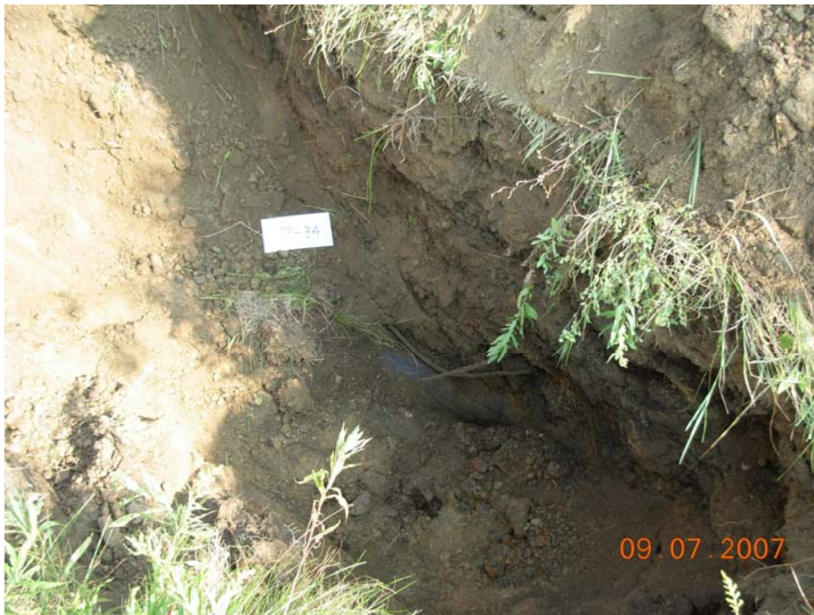
Test Pit 34 with water main exposed
