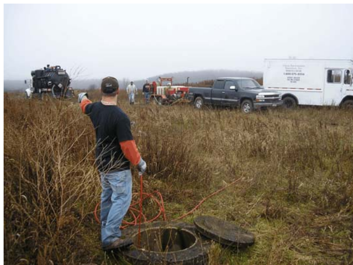
Flushing Leachate Pipes
