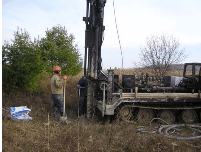
Drilling MW-2 (West Side of Landfill)
