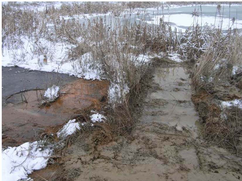
Ditch Excavated to Direct Tank Overflow to Pond
