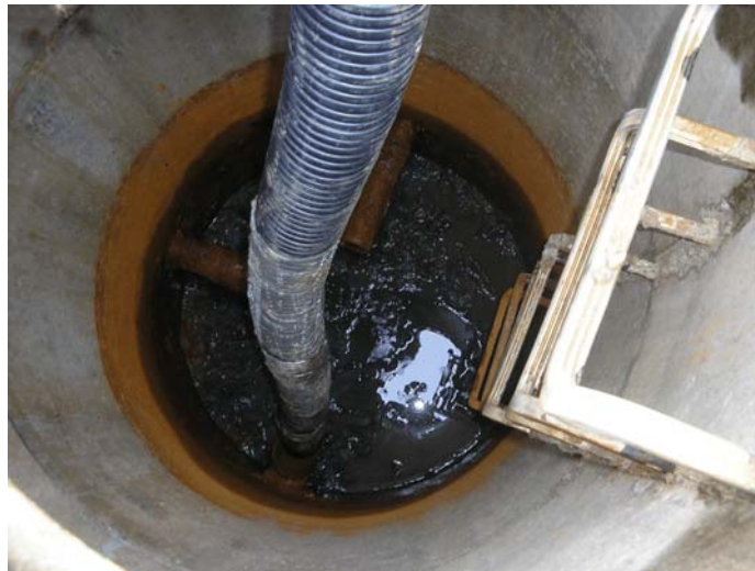
Removing Sediment From Manhole
