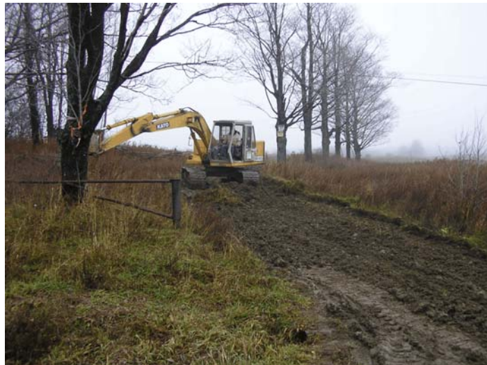
Excavator Fixing Access Road
