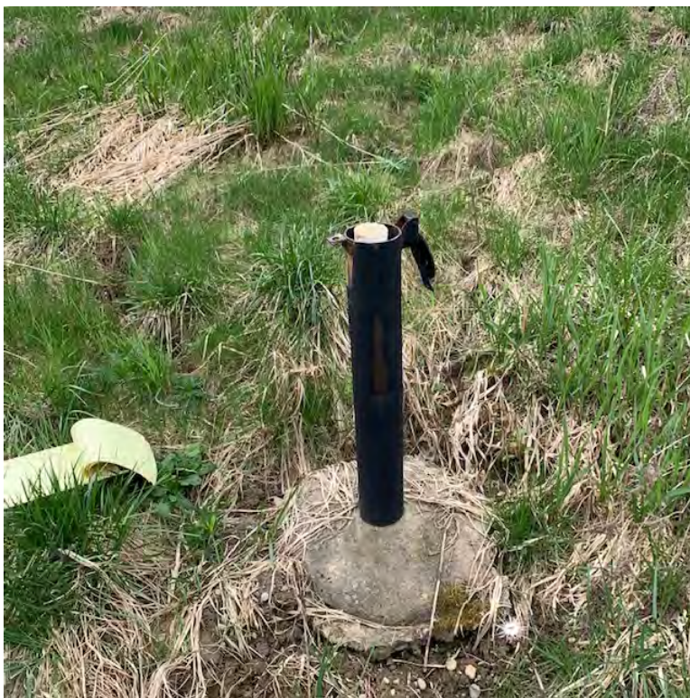
Photo 10 – MW-2S(R) found uncapped and unlocked.
