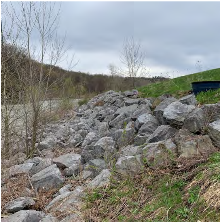
Photo 12 – View upstream from lift station manhole with visible trees and shrubs growing in rip rap.
