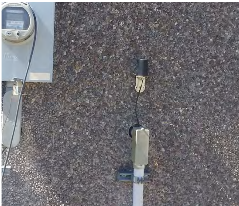
Photo 14 – Treatment Building – Alarm cell antenna location and mount susceptible to vandalism.
