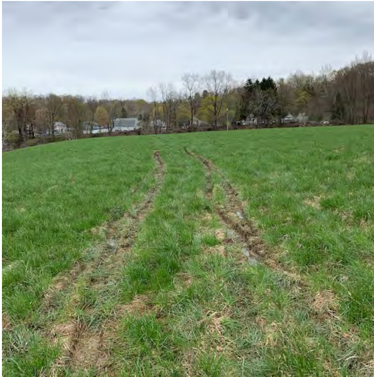
Photo 5 – Truck ruts on cap.
