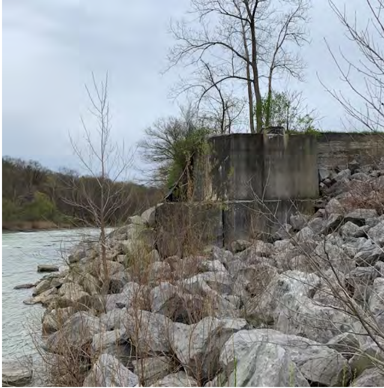
Photo 13 – View upstream from rip rap at concrete wall beginning showing trees and shrub growth.
