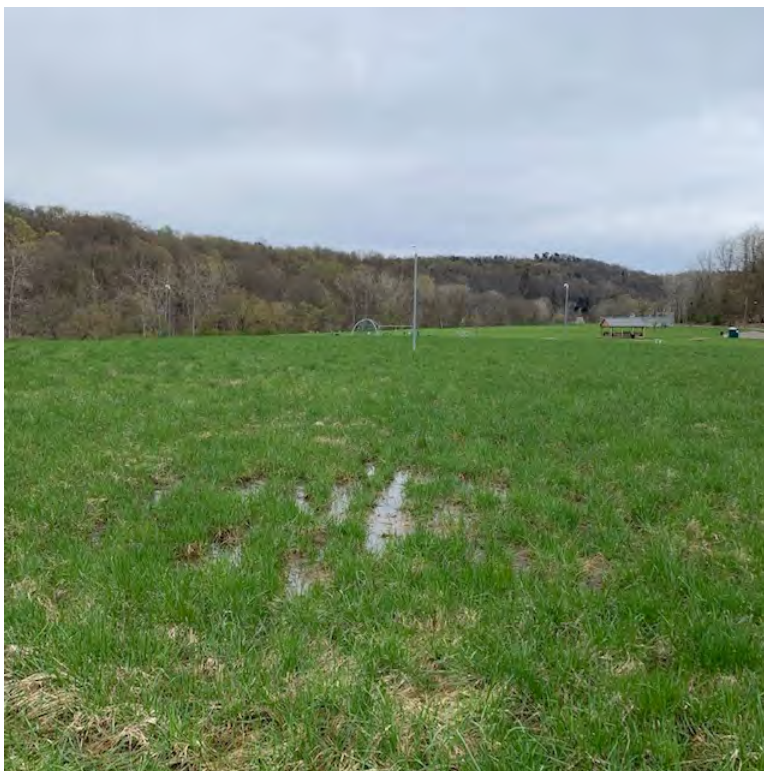
Photo 8 – Ponding water on cap.
