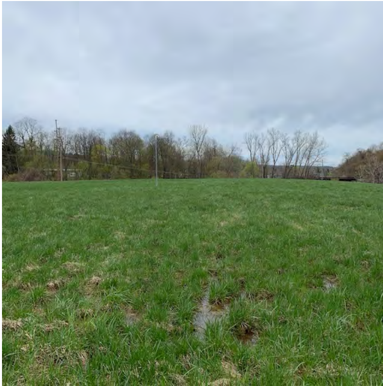
Photo 9 – Ponding water on cap.
