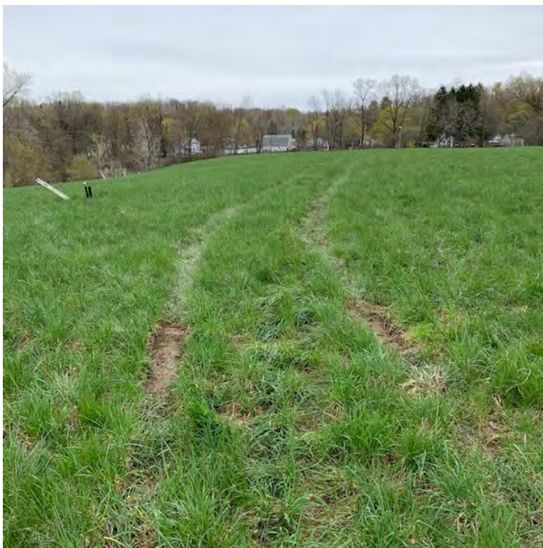
Photo 4 – Truck ruts on cap.
