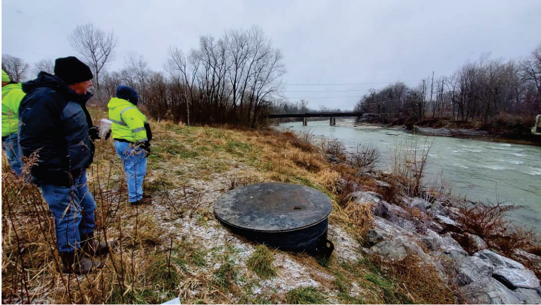
View of riprap and manhole for leachate/groundwater collection.
