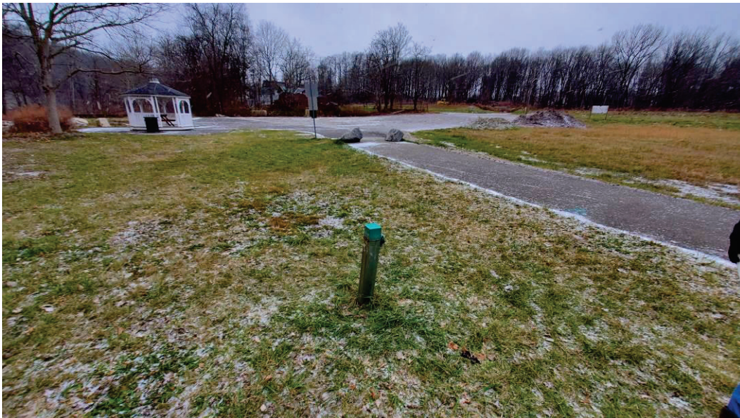
View of MWFP-2S which had been bent earlier in the year due to equipment operation. The bend has since been repaired.
