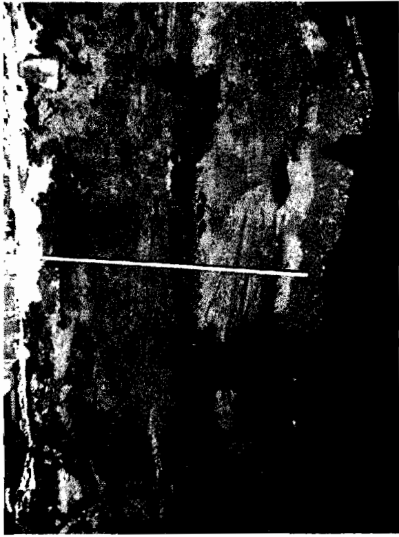
Plating Vat area excavation showing layers of high chromium contaminated soil along east side of excavation.
