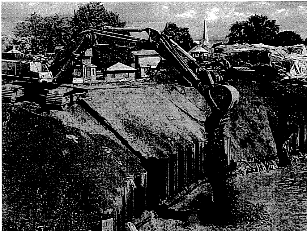
14. Backfilling: Groundwater treatment of 3,056,000 gallons was completed and backfilling was begun.
