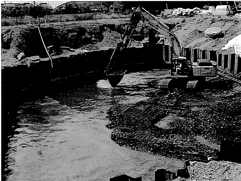
8. Hazardous Soil Excavation: Continuing excavation of soil below groundwater. (Note Yellow water)
