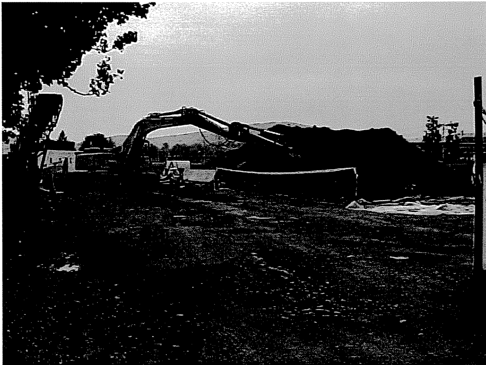
12. Hazardous Soil Excavation: Hazardous Soil staging pad.
