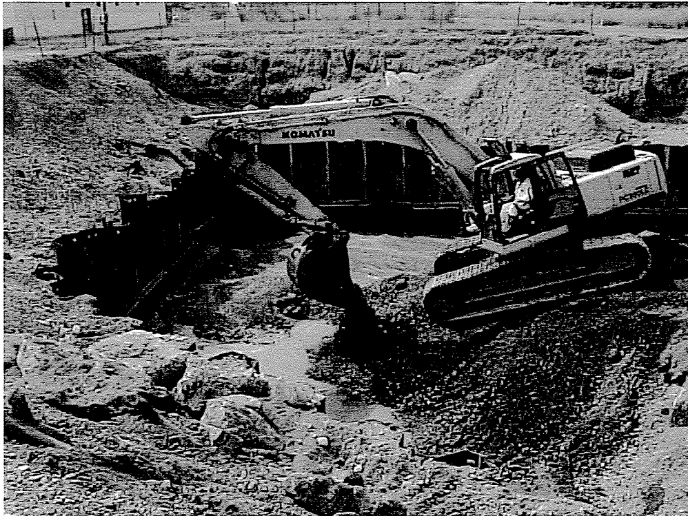
7. Hazardous Soil Excavation: Start of excavation of soil below 18' bgs.
