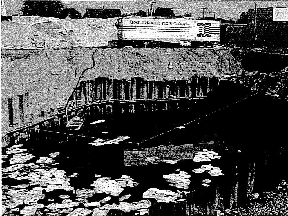
13. Groundwater Treatment: Groundwater Treatment Unit Trailer w/ submersible pump suspended in center of excavation.
