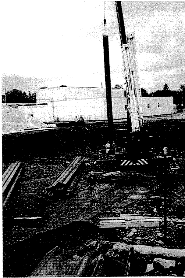
3. Shoring Installation: Setting sheets in place.
