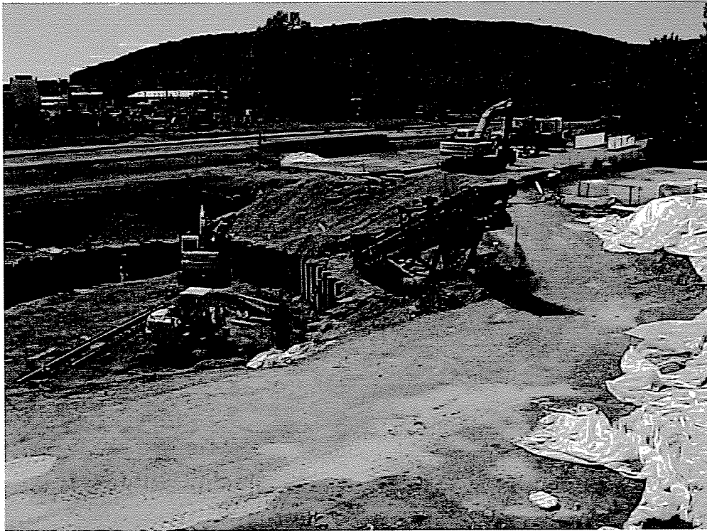
5. Shoring Installation: Overview of excavation and anchor installation.
