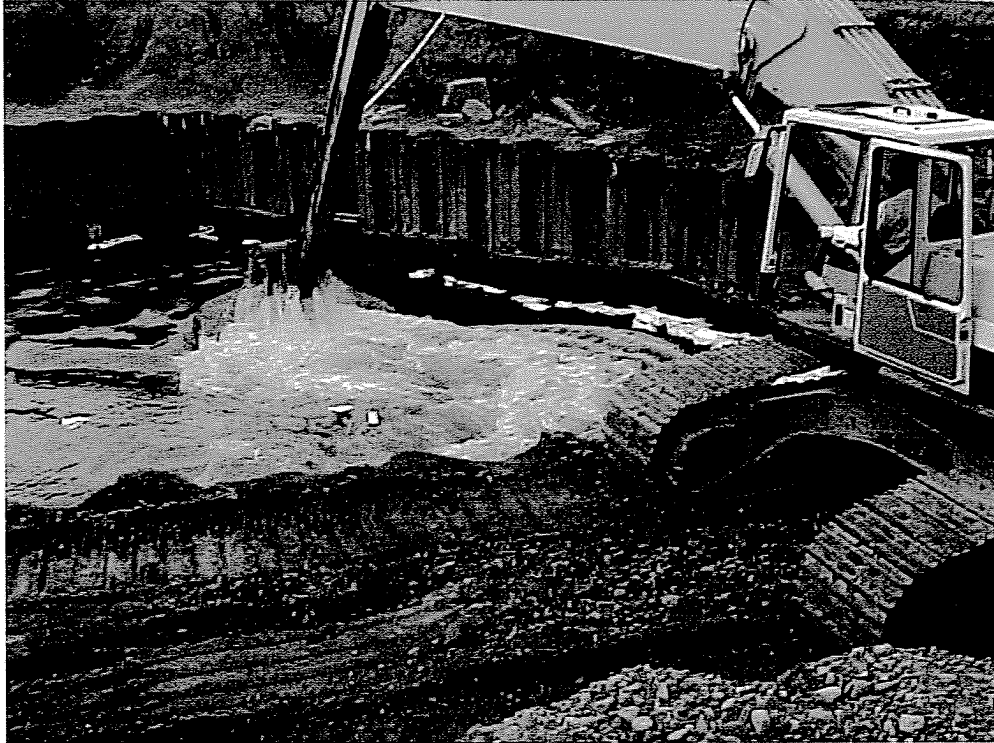
11. Hazardous Soil Excavation: Excavating through chromium contaminated groundwater.
