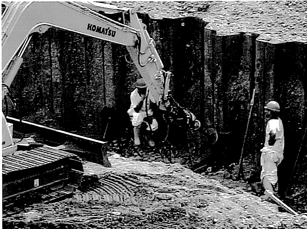
6. Shoring Installation: Installing anchors into shoring.
