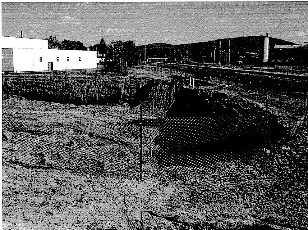
2. Non-Hazardous Soil Excavation: Initial 15 foot cut in area of shoring to remove uncontaminated soil from the work area.
