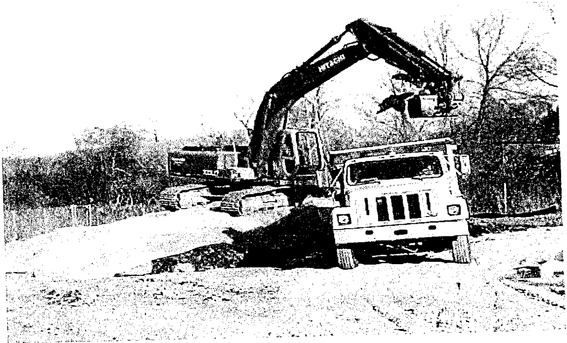
Loadout of Stockpiled Soil from Area C2 and 03
