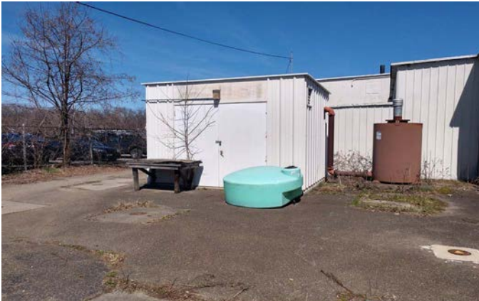
Asphalt cap at AST/UST Area:
