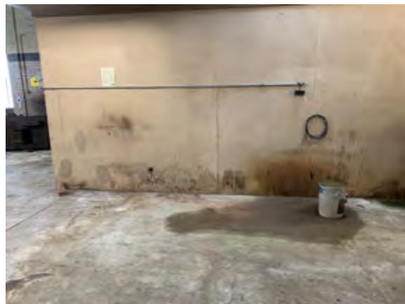
Photograph 4: Evidence of water damage
