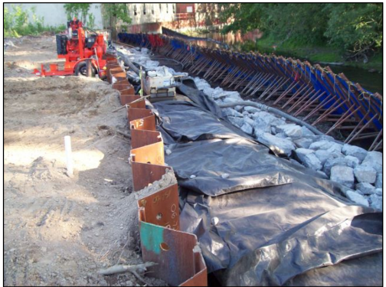
Sheet pile construction along riverbank
