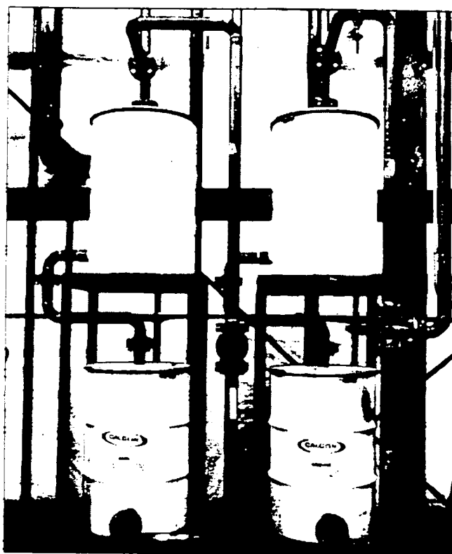
Four VentSorb units at a chemical plant are installed to operate in series and in parallel. More than 25 odorous and/or toxic vapors are controlled by 80 VentSorb units at this plant.
