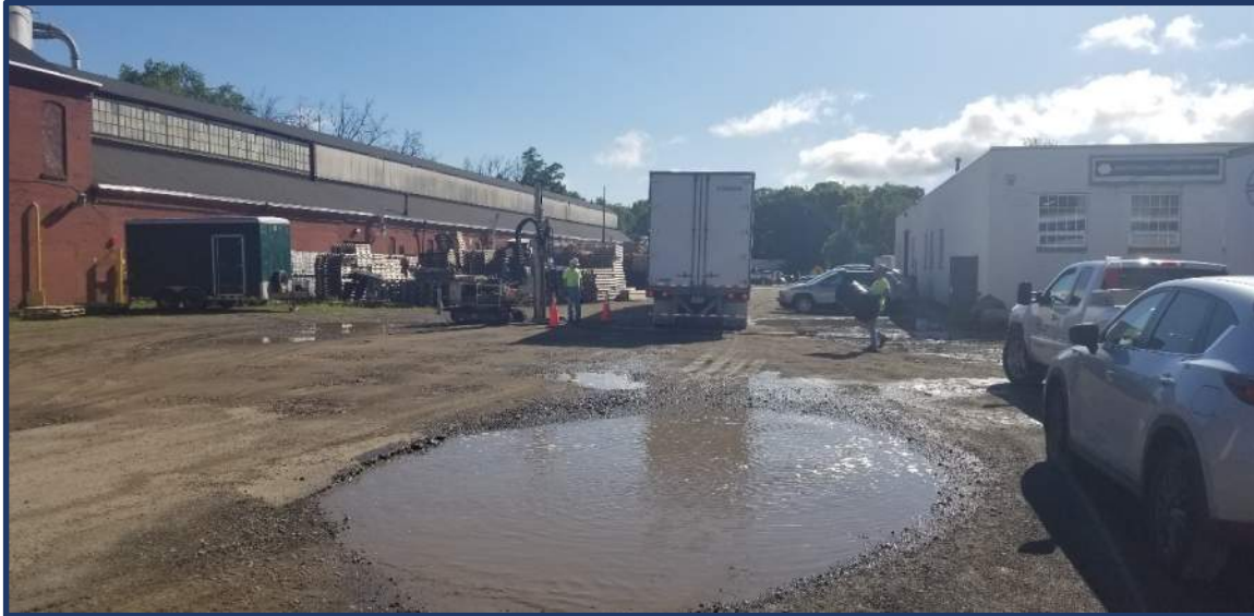
Photo 5 – Injection of chemicals
