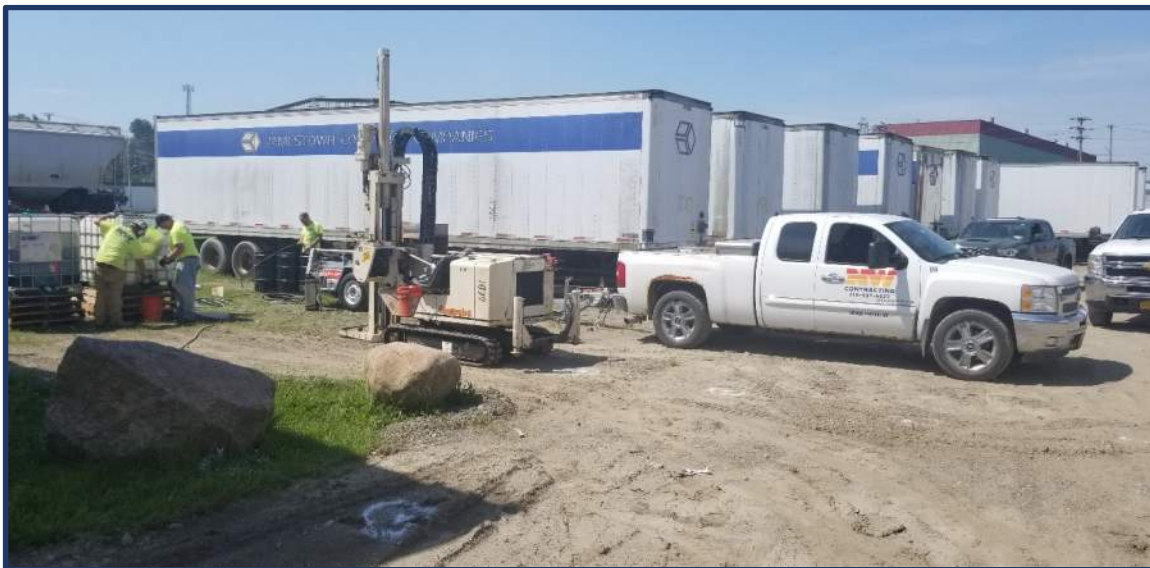
Photo 4 – View of injection and staging area.
