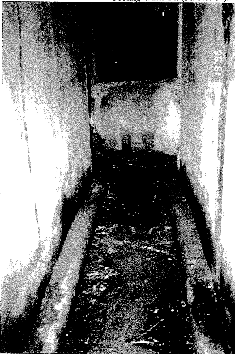
Photograph 7 - Slight peeling of tar-like coating of the wall in the Vaughn Cooling Water Pit (Pit No. 14).
