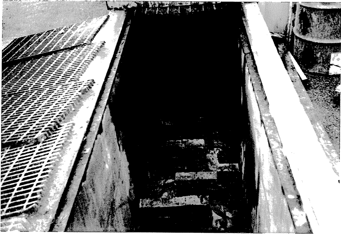
Photograph 13 - View of the Serpentine Outfall (Pit No. 29) which discharges to the POTW sewer line.
