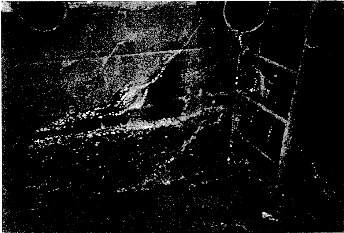
Photograph 3 - Walls and floor of the Shark Pit (Pit No. 8) coated with oil and grease. Also, groundwater infiltrating through several cracks.
