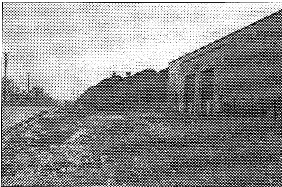
Outside of building, looking east
