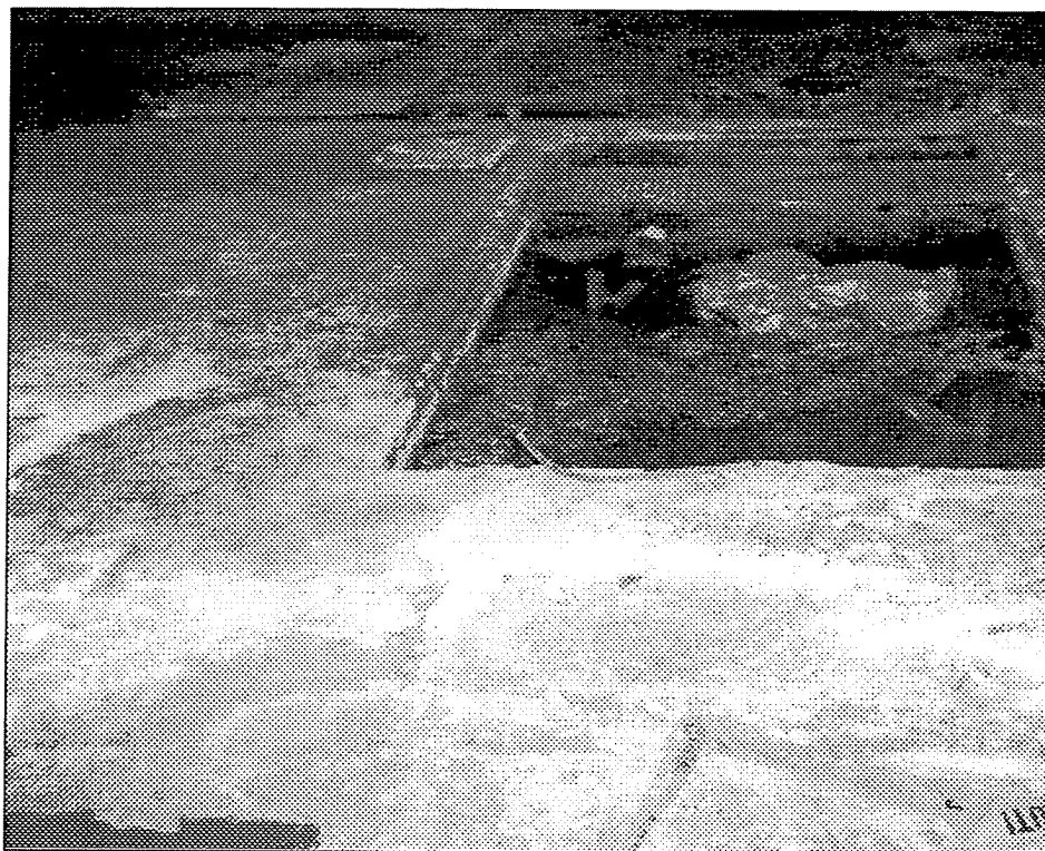
Hydrogen annealing floor pit in East Production Room
