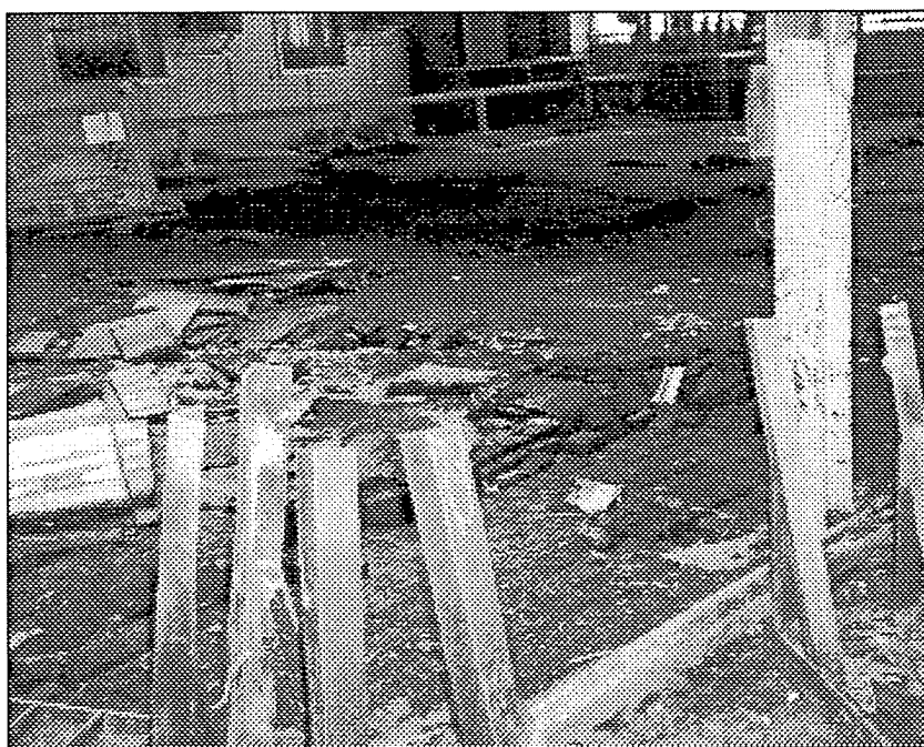
Wood block flooring in Drawing Oil Area of East Production Room
