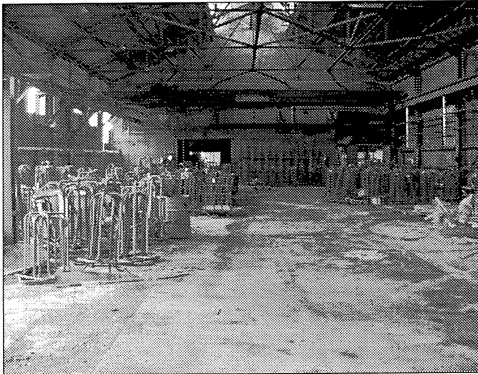
East Storage Room looking west
