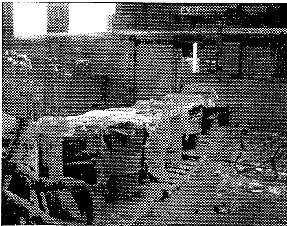
Open drums in East Storage Room with scrap metal
