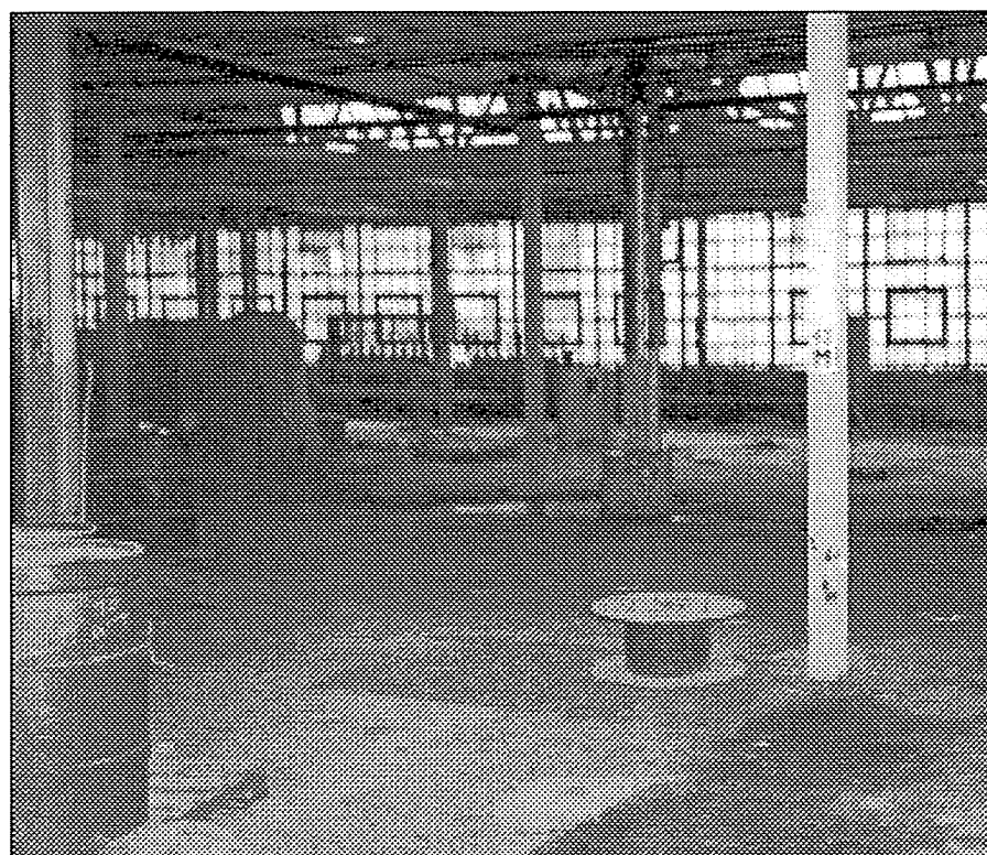
North wall of West Production Room
