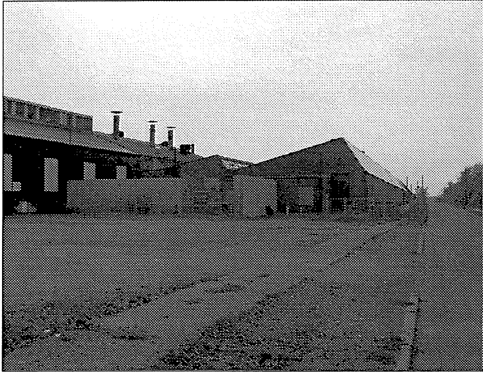
North side of building, looking west
