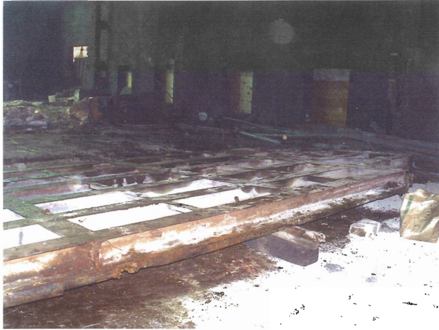
Photo 15. Tank bottom support super structure
