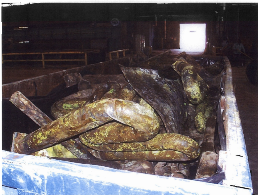
Photo 12. Contaminated steel tank components in roll-off awaiting disposal
