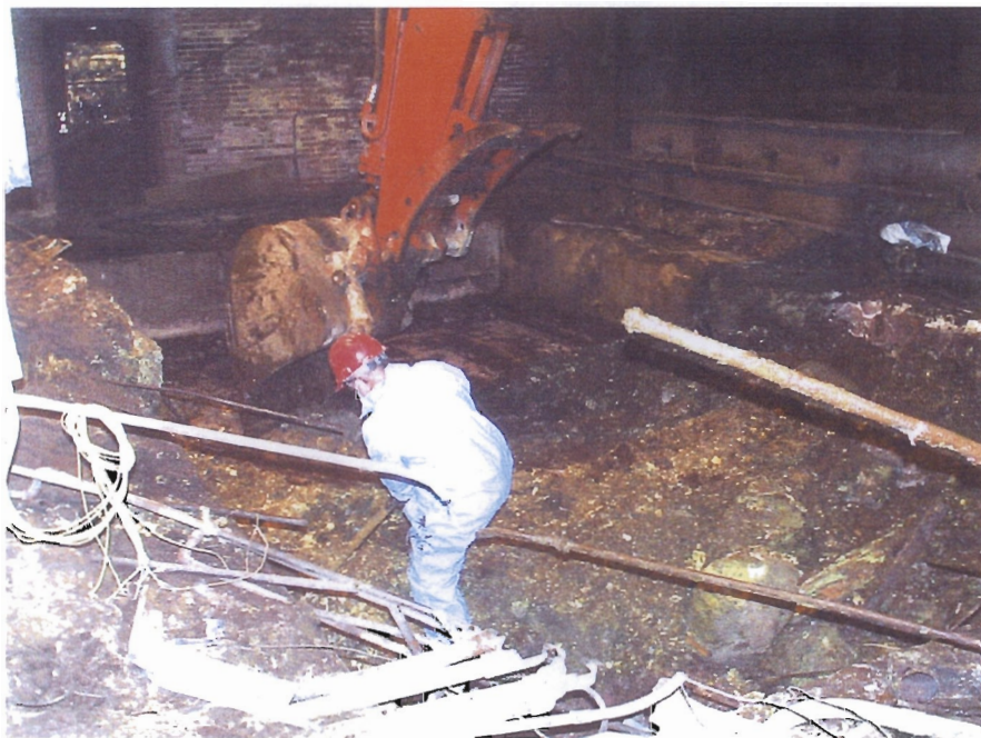
Photo 14. Residuals clean-up in tank pit
