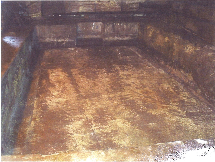
Photo 17. Tank pit following final clean-out - looking east
