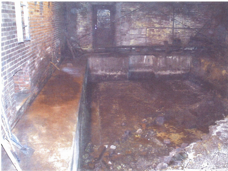
Photo 16. Tank pit looking east
