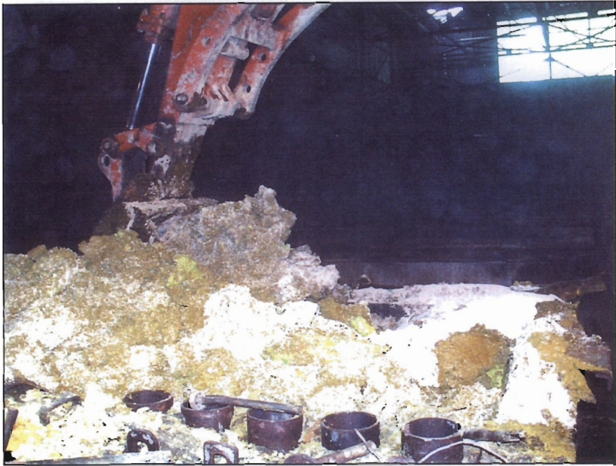
Photo 1. Mixing of clay absorbent w/ liquefied kolene residuals
