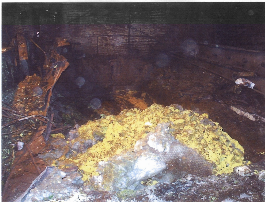
Photo 11. Insulating brick residue stockpiled for disposal
