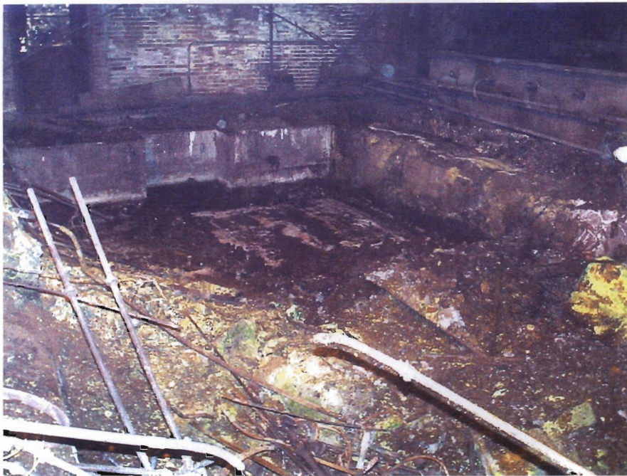
Photo 13. Exposed tank pit looking east
