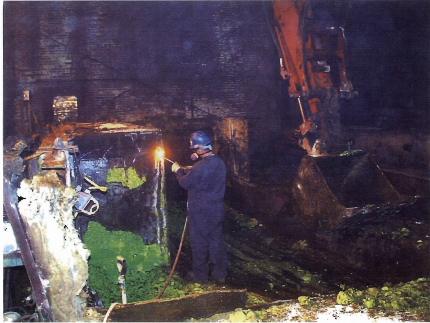
Photo 9. Mixing compartment removal
