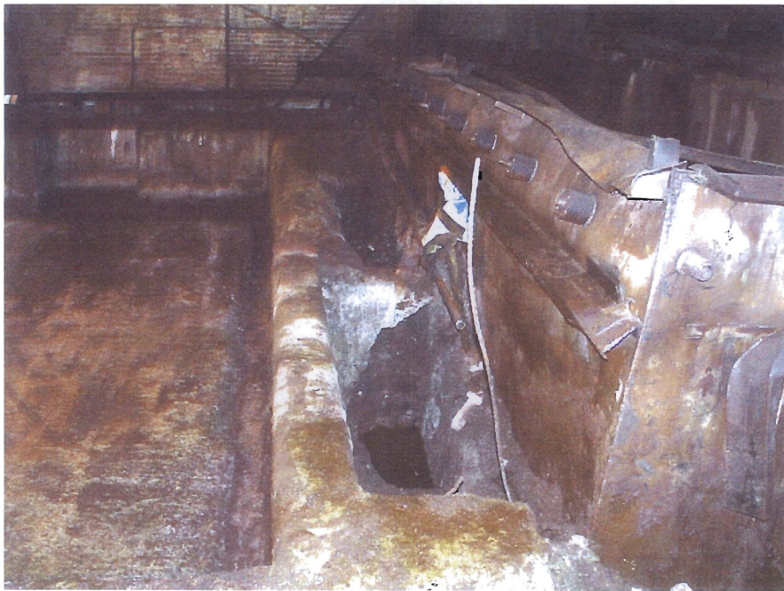
Photo 18. Tank pit and adjacent south pit after final clean-out
