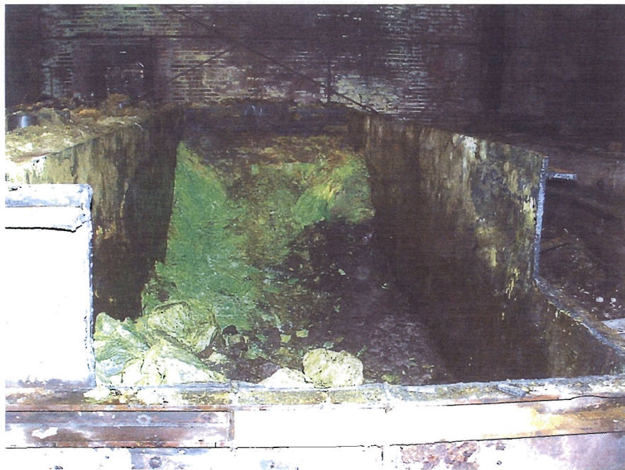
Photo 6. Solidified Kolene in process portion of tank (looking east)
