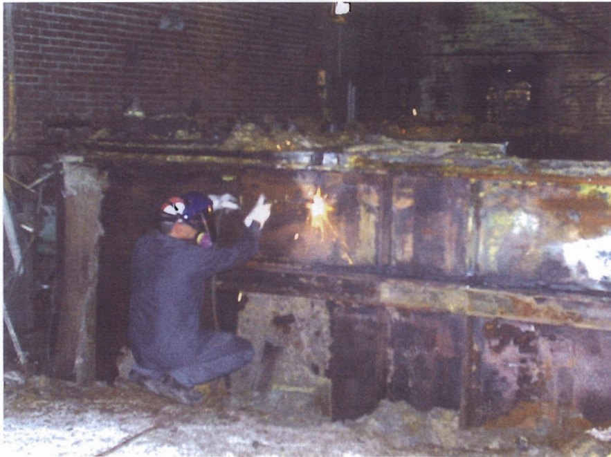
Photo 4. GEI initiating cutting of west wall of inner tank shell
