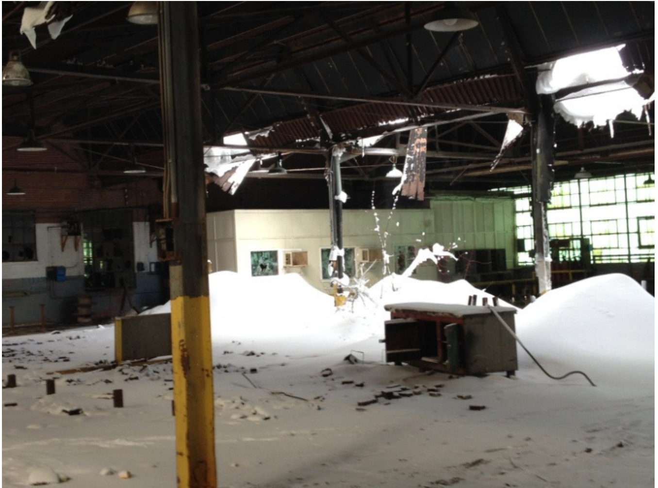
Photo 10: Failed sawtooth metal roof deck near east office
