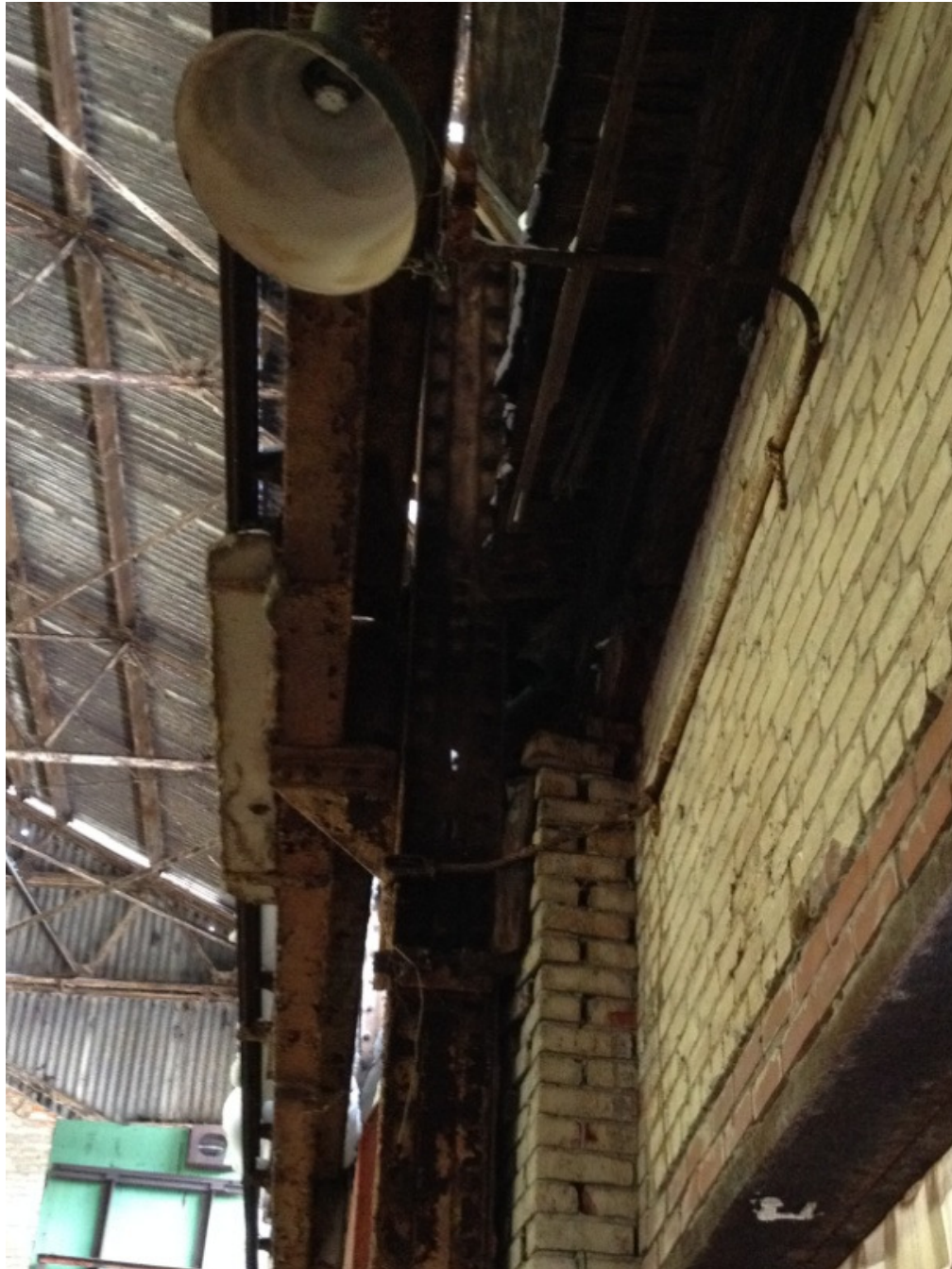
Photo 20: Curved column & rust through holes in web
