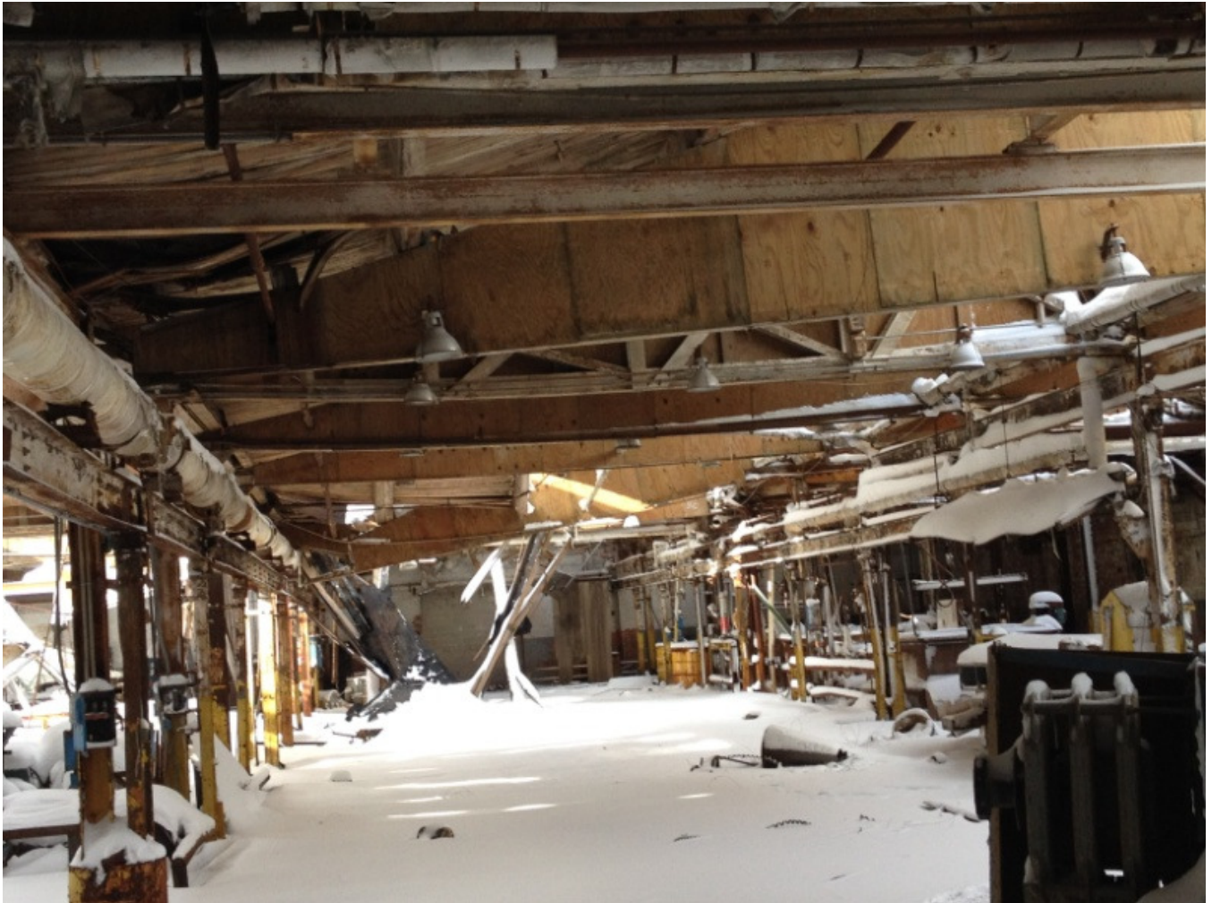
Photo 16: Bowed and collapsed plywood faced trusses
