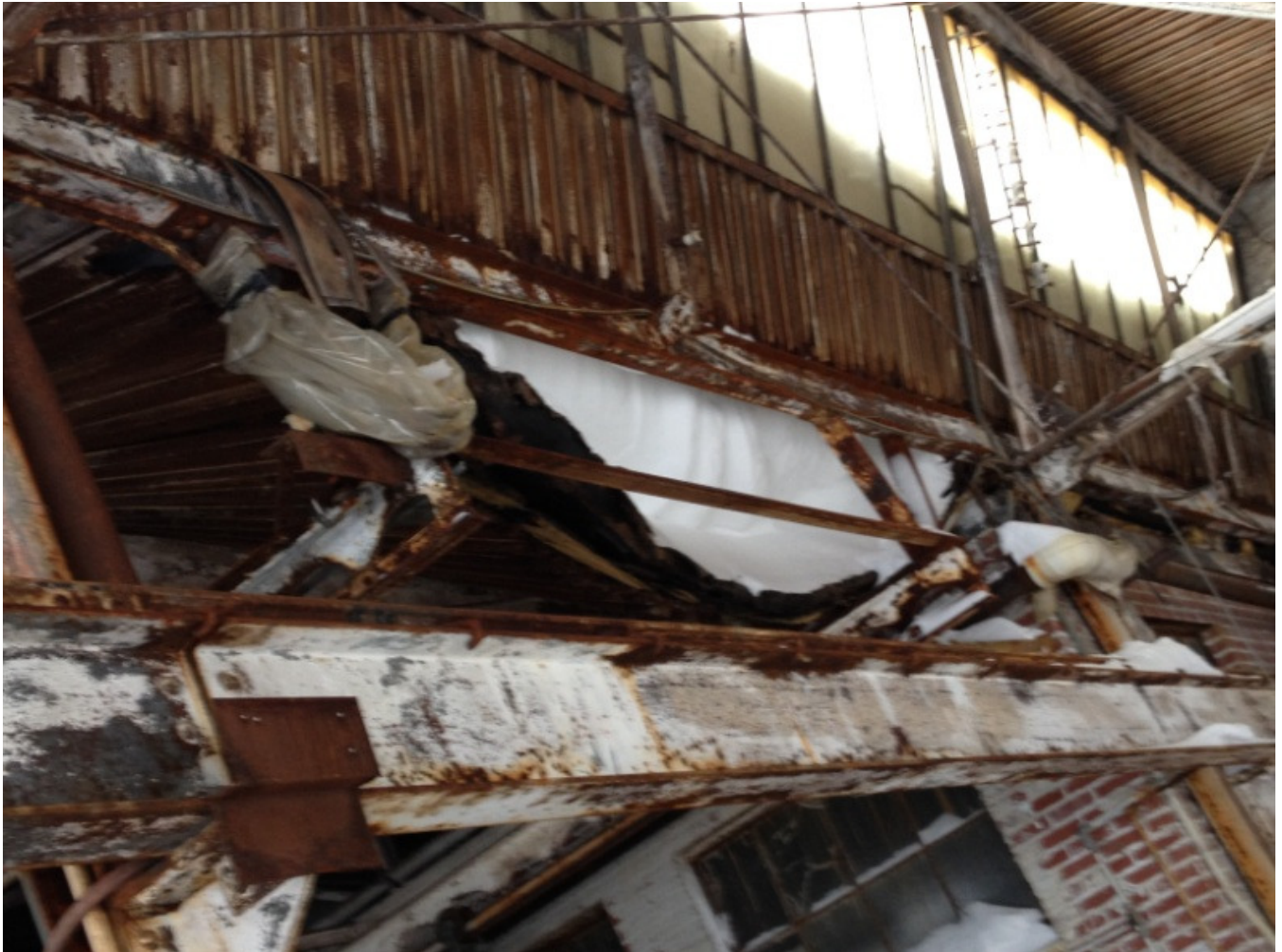
Photo 12: Failed metal roof deck due to snow load
