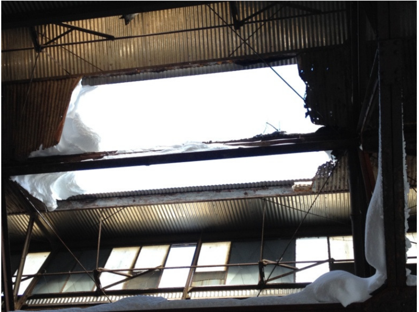
Photo 4: E. warehouse failed monitor deck & snow drift
