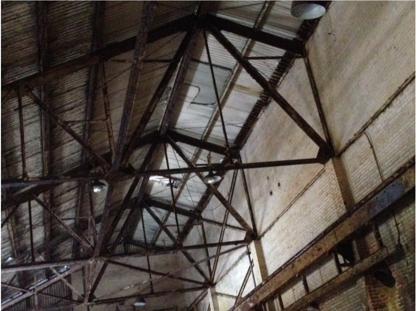
Photo 5: East Pickling area brick masonry and steel roof trusses
