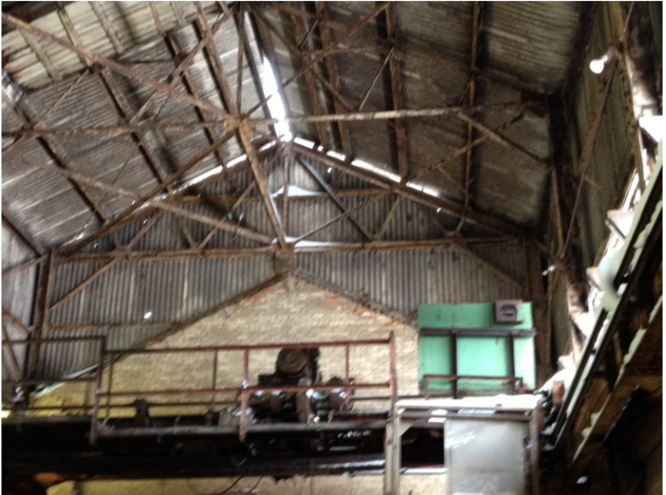
Photo 17: Steel trusses and metal deck form high roof
