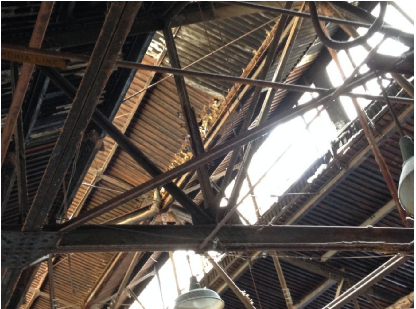
Photo 6: Southerly high bay deck with rust through holes
