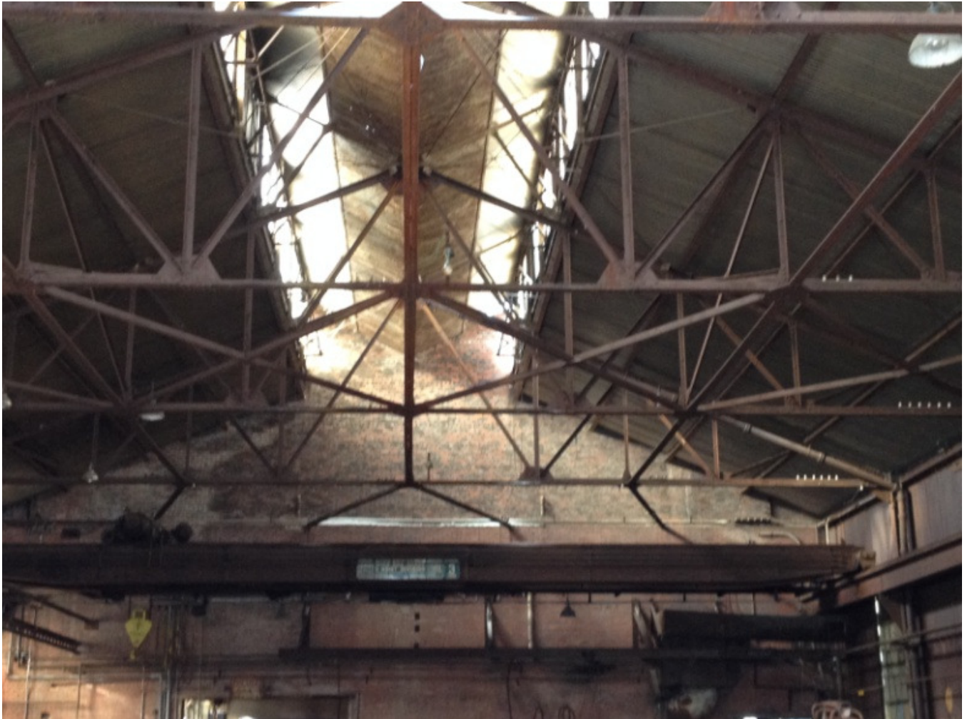
Photo 2: E. end roof trusses & bridge crane
