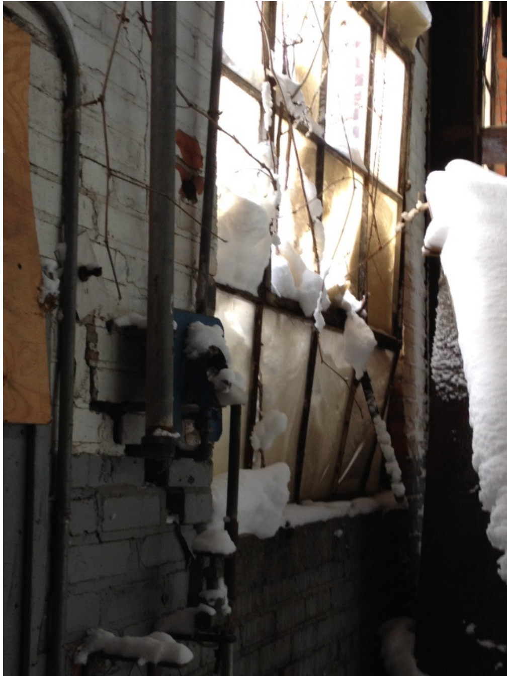
Photo 8: Southerly brick wall bowed & cracked
