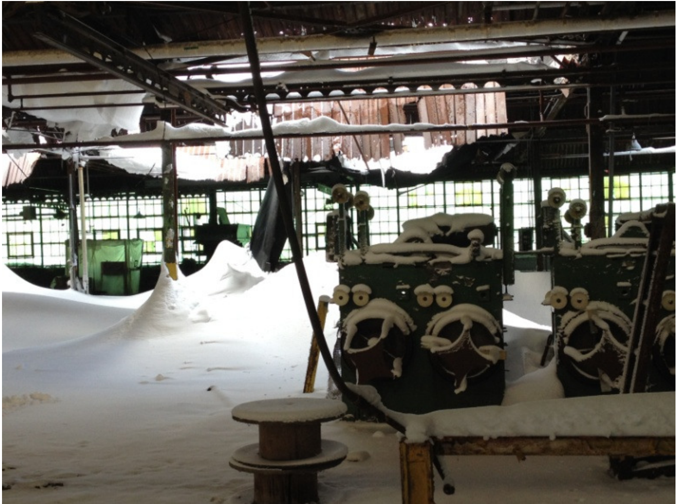
Photo 7: Northerly part with collapsed metal roof deck
