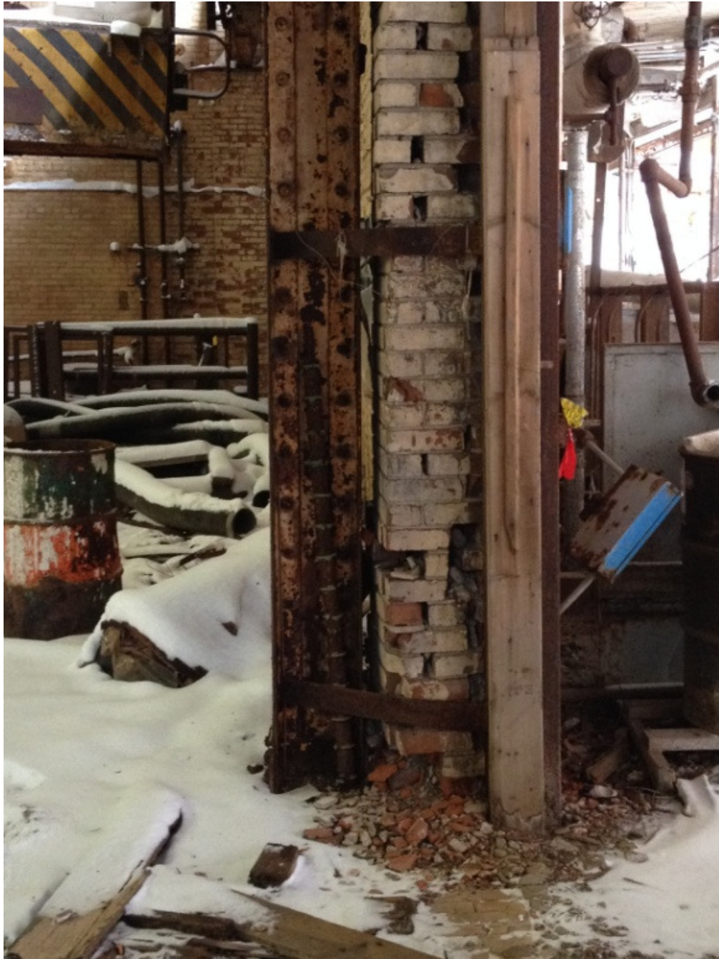
Photo 19: Failing brick masonry wall with large structural cracks
