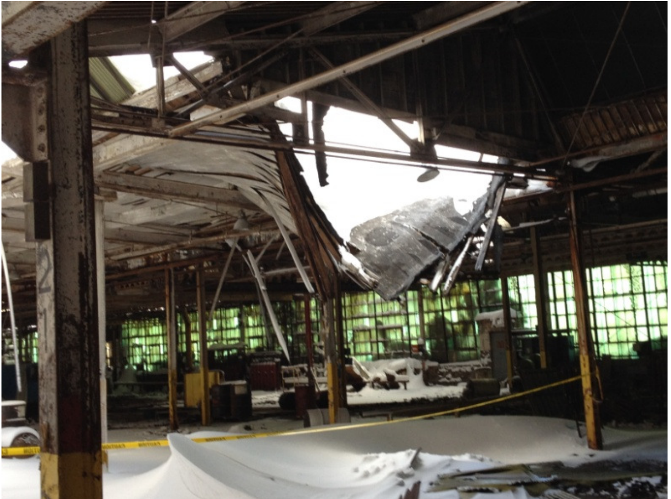
Photo 13: Failed flat roof area at metal to wood transition
