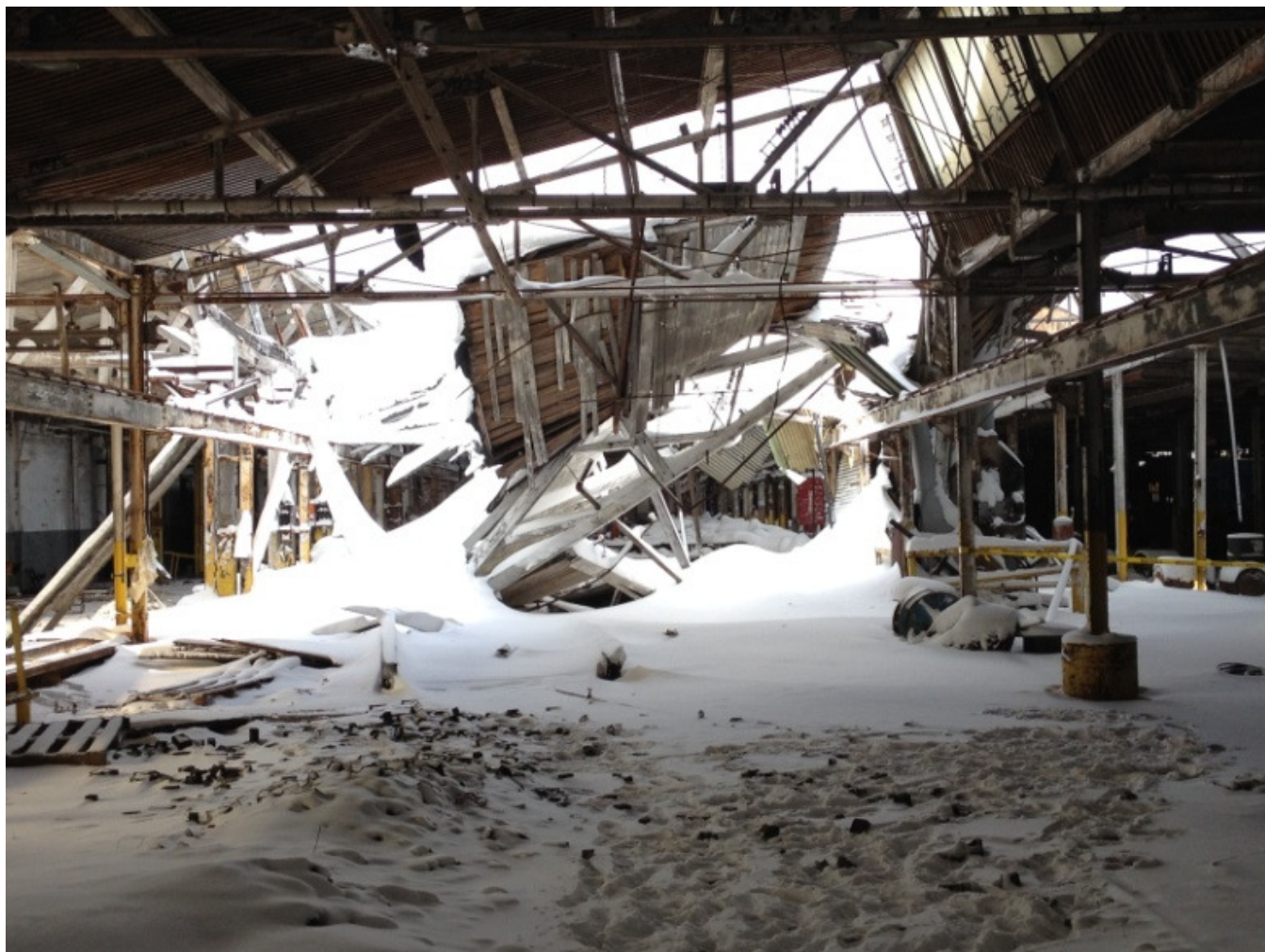
Photo 11: Collapsed transition from metal wood framing
