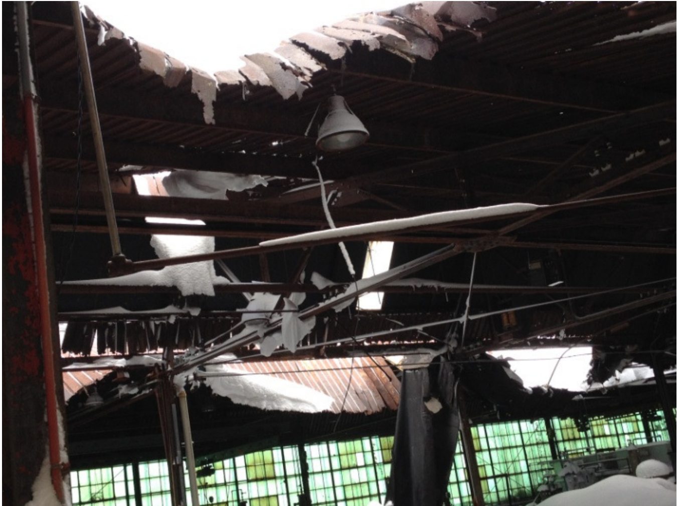
Photo 9: Failed sawtooth metal roof deck multiple bays
