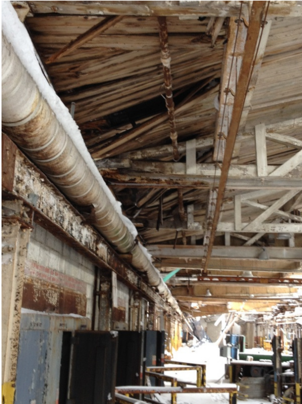
Photo 15: Failed wood deck from rot
