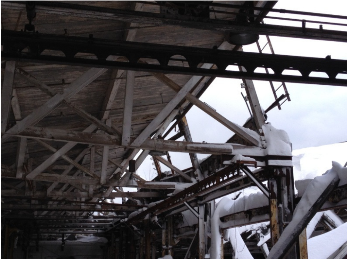
Photo 14: Collapsed wood framed sawtooth roof
