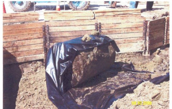
UST removed from location and placed on plastic sheeting, looking north.
