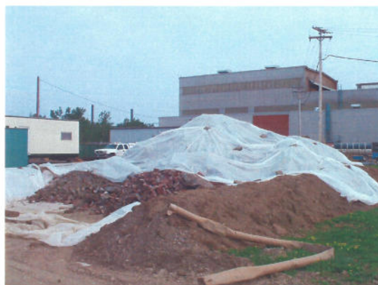
Oily contaminated soil stockpile placement on plastic sheeting and within soil berms, looking northwest.
